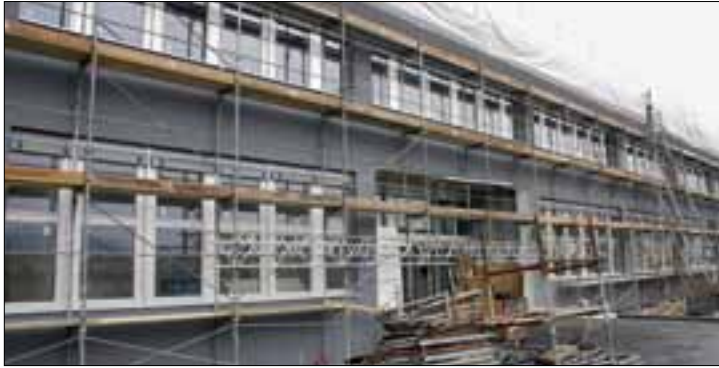
Final construction stage of the Riverside Campus building, 2010.
