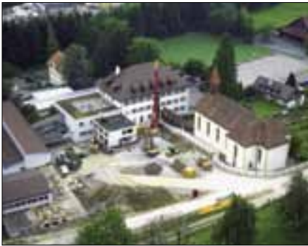
Initial phases of construction on the new Middle School, July 2009.
