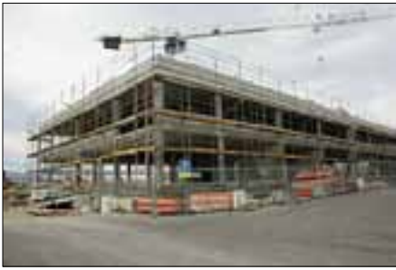
Construction of the Riverside Campus building, October 2009.
