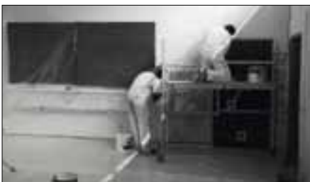
Painting the Walterswil classrooms, 1997.
