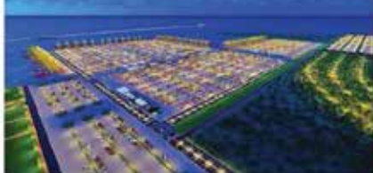
Construction site of Vadhvan Port
