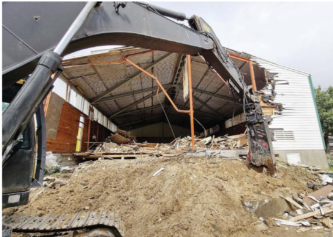
Onslow College's former Rec Centre being demolished. Photo: Supplied.
