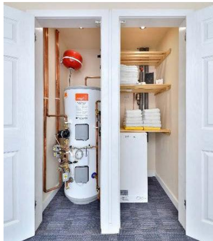
Sunamp heat batteries can help with DHW where internal space is limited
