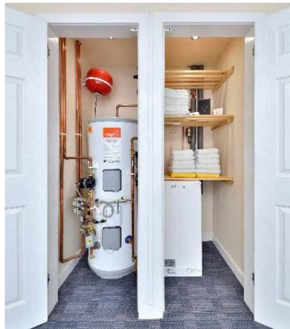
Sunamp heat batteries can help with DHW where internal space is limited
