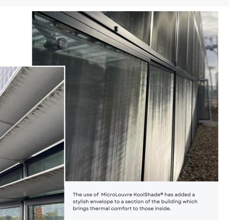
It is a highly efficient and versatile woven metal fabric. Its micro-louvres are set at specific angles to stop solar heat gain and glare, and is non-combustible.
