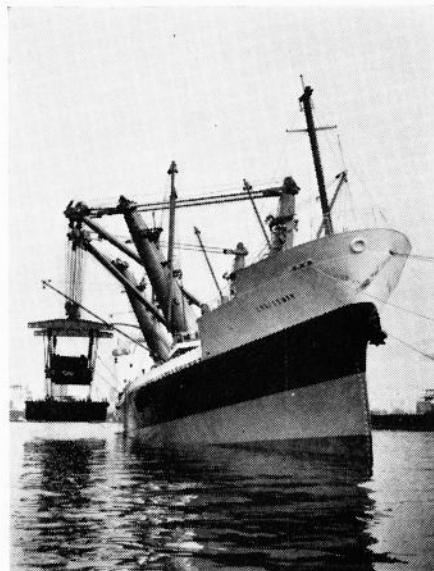
Test load of 550 tons on the two Stülcken derricks. The list is not excessive
