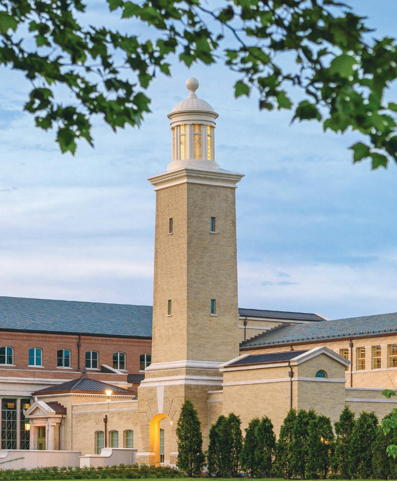
Matthew and Joyce Walsh Family Hall of Architecture on the campus of the University of Notre Dame in Notre Dame, Indiana
