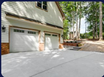
Attached 2-Car Garage
