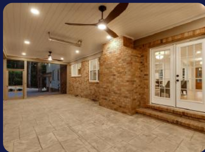
Covered Heated Patio
