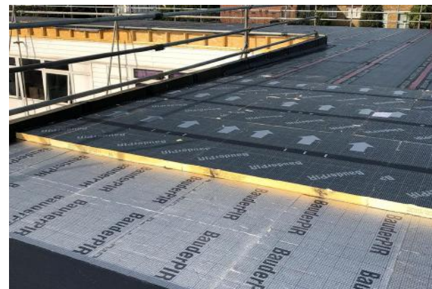
Insulation laid over a flat roof forming part of the building envelope (source: Bauder)
