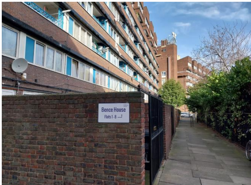
(left) The Pepys Estate with Bence House in the foreground (right) Axonometric view of the Pepys Estate and adjoining housing blocks
