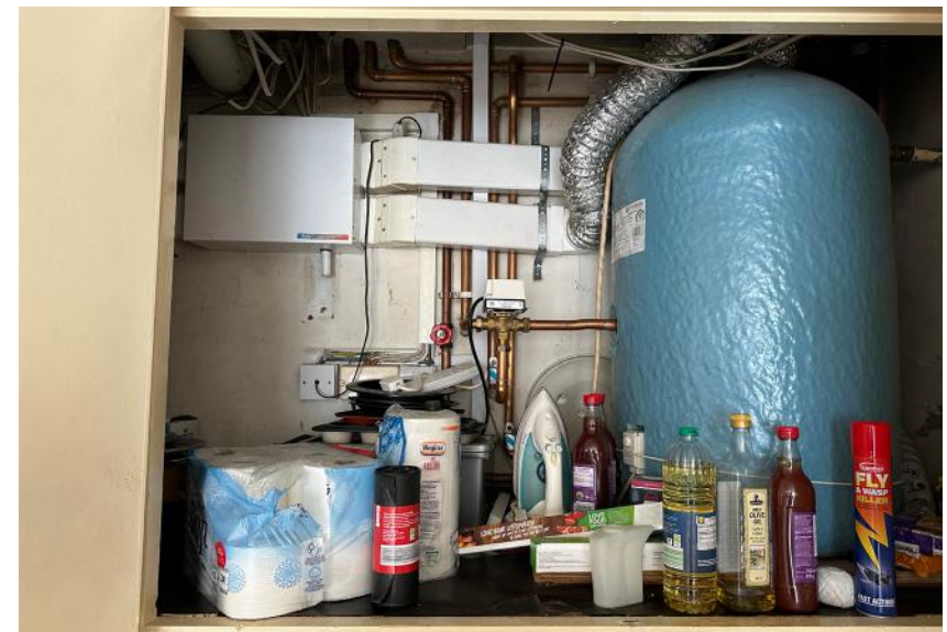
(far left) Type A flat, lower level floor plan; (left) Type A flat, upper level floor plan; (above left) Gas boiler in kitchen on lower level with flue to private garden; (above right) cold water header tank in bedroom service riser with MVHR ducts; (below) domestic hot water storage cylinder and MVHR unit within kitchen service riser.
