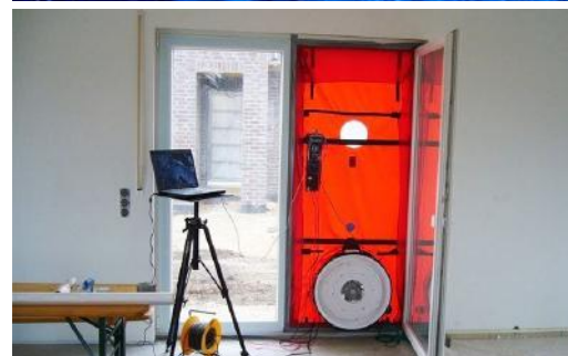
In a Blower Door airtightness test, a powerful fan is mounted to the front door of the property to create negative pressure inside the home. This causes air to flow in through any gaps, cracks, or openings.
