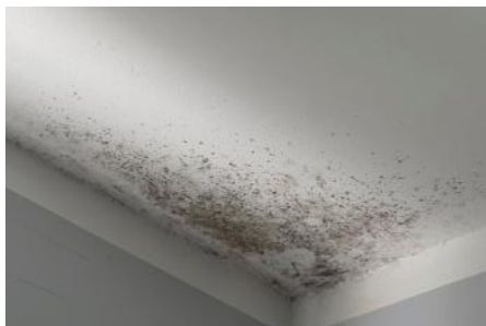
Black mould on living room ceiling under area of communal roof of 6th floor escape balcony
