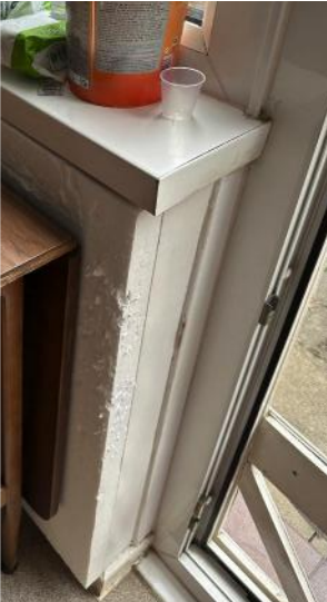
DIY internal insulation to address thermal discomfort in winter
