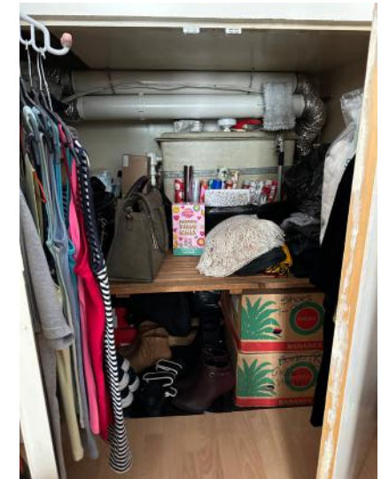
(far left) Type A flat, lower level floor plan; (left) Type A flat, upper level floor plan; (above left) Gas boiler in kitchen on lower level with flue to private garden; (above right) cold water header tank in bedroom service riser with MVHR ducts; (below) domestic hot water storage cylinder and MVHR unit within kitchen service riser.
