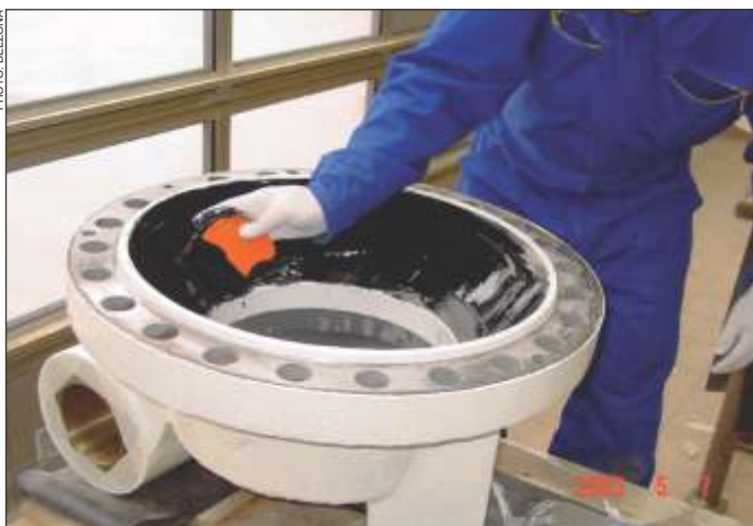
Application of Belzona 2141 (ACR-Fluid Elastomer) on Pelton turbine nozzle head.
