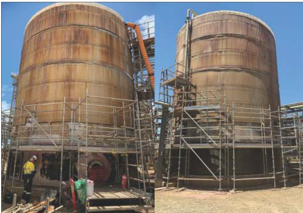
Figure 3. Stainless steel feed tank repaired and protected with Belzona SuperWrap II.
