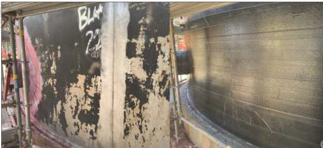
Figure 1. Composite wrap system curbs corrosion under insulation at nickel mine.
