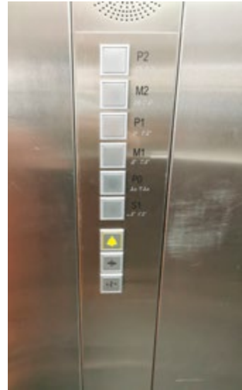
Ascensor B / Elevator B
