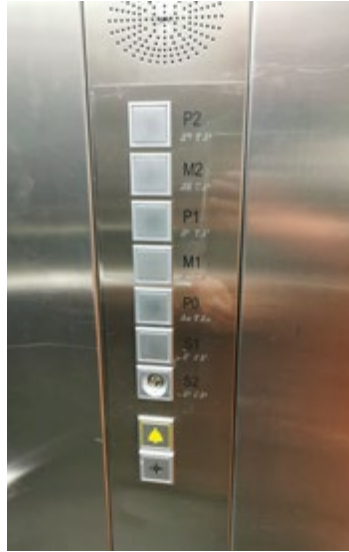
Ascensor C / Elevator C
