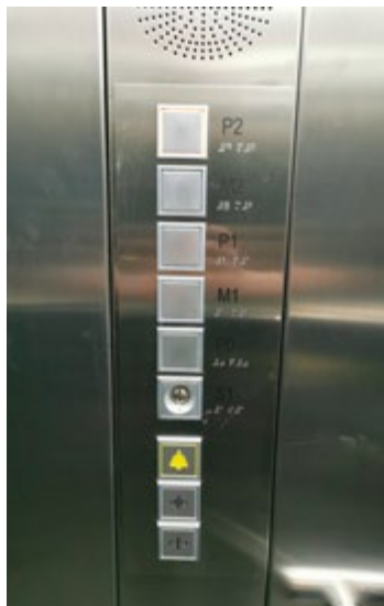
Ascensor D / Elevator D
