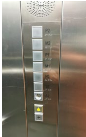
Ascensor C / Elevator C
