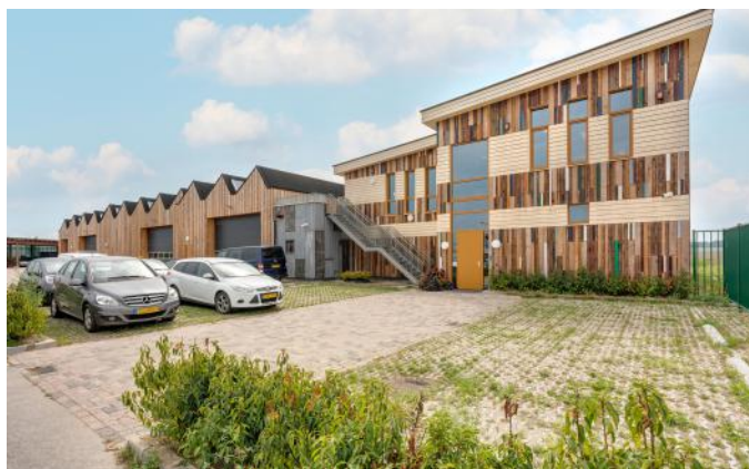
Nieuwkoop: Ruben Visser, Orga Architect
