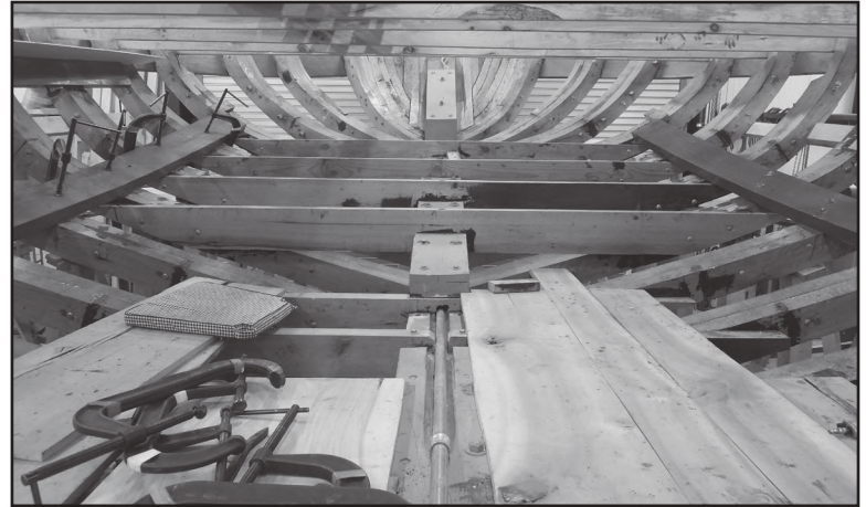
Bilge stringers, floor boards, keelson, October 2014.
