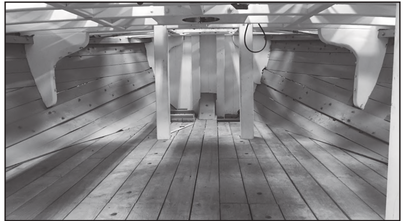
Knees, ceiling planks, deck beams, November 2017
