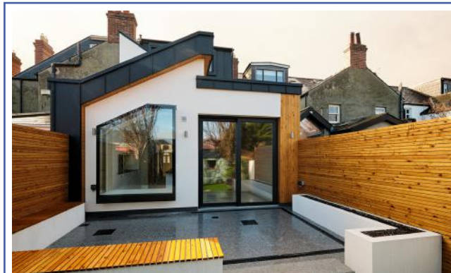
Cliftonville Av, Dublin 9
