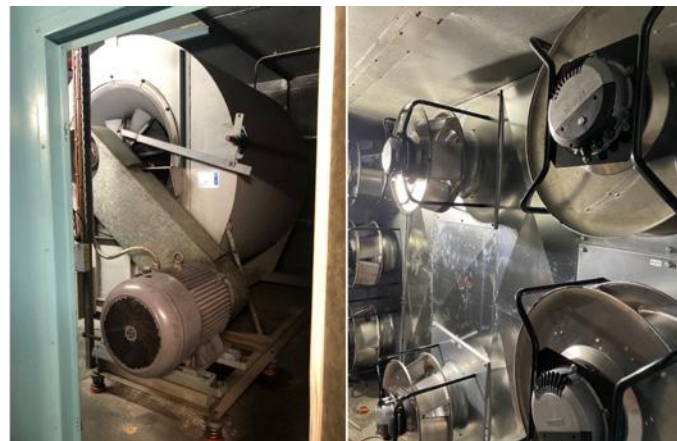
Figure 4: Before and after photos of the EC fan upgrade for AHU 4.
