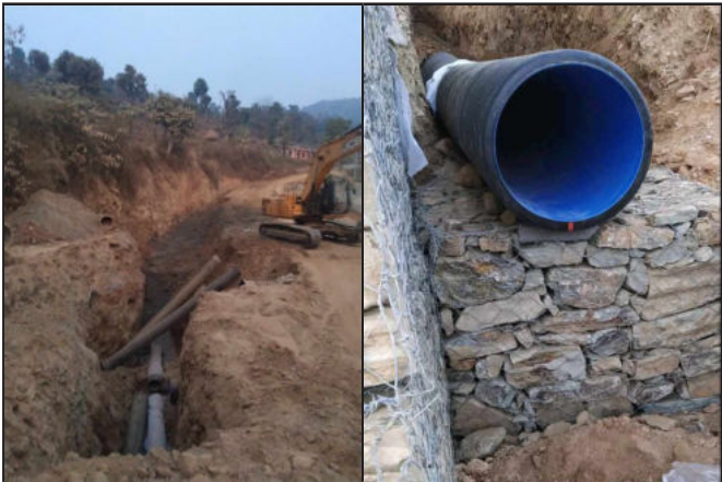
Figure 7: Construction of gravel trench and perforated pipe below side drain and its outlet pipe across road
