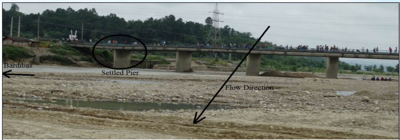
Fig. 5 (b) Pier of Ratu Khola Bridge settled on 13 Aug, 2014
