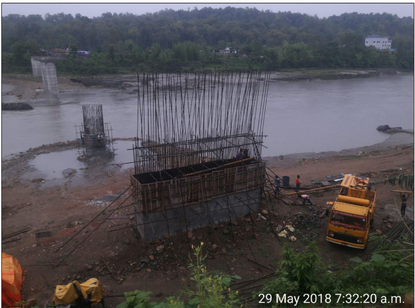
Figure 3: Foundation and Substructure Works
