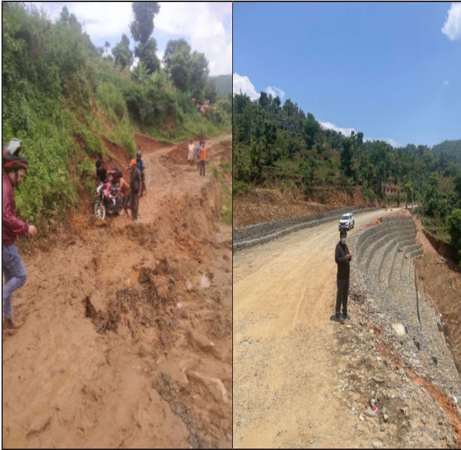
Figure 13: Road condition at Kokhe Aahale in June 2022 (left) and road condition after application of mitigation measure in May 2024 (right).
