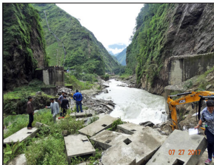
Fig.8-(a) Larcha Arch bridge collapse due to sudden fall of rock from hill side (2017-7)
