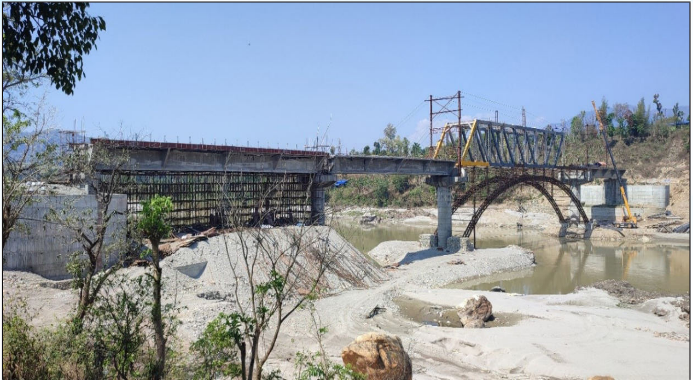
Figure 4: Construction work of PSC and Truss Span
