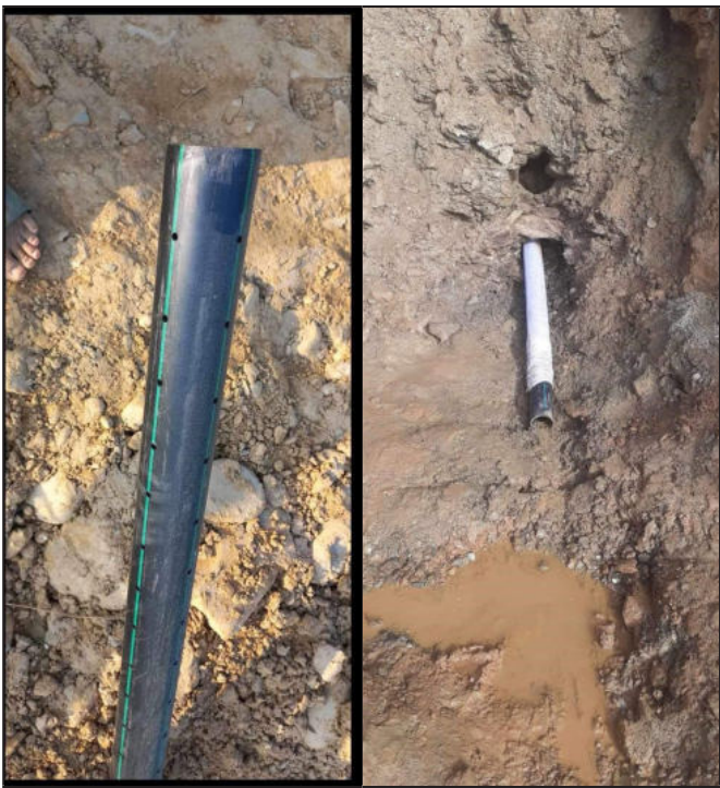
Figure 10: Perforated HDPE pipe and horizontal drainage in drilled hole for sub-surface drainage.
