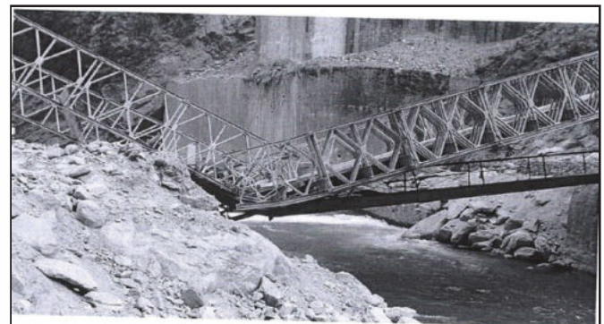
Fig.4(d). Larcha Bailey bridge failure during erection (in 2018-02-20)
