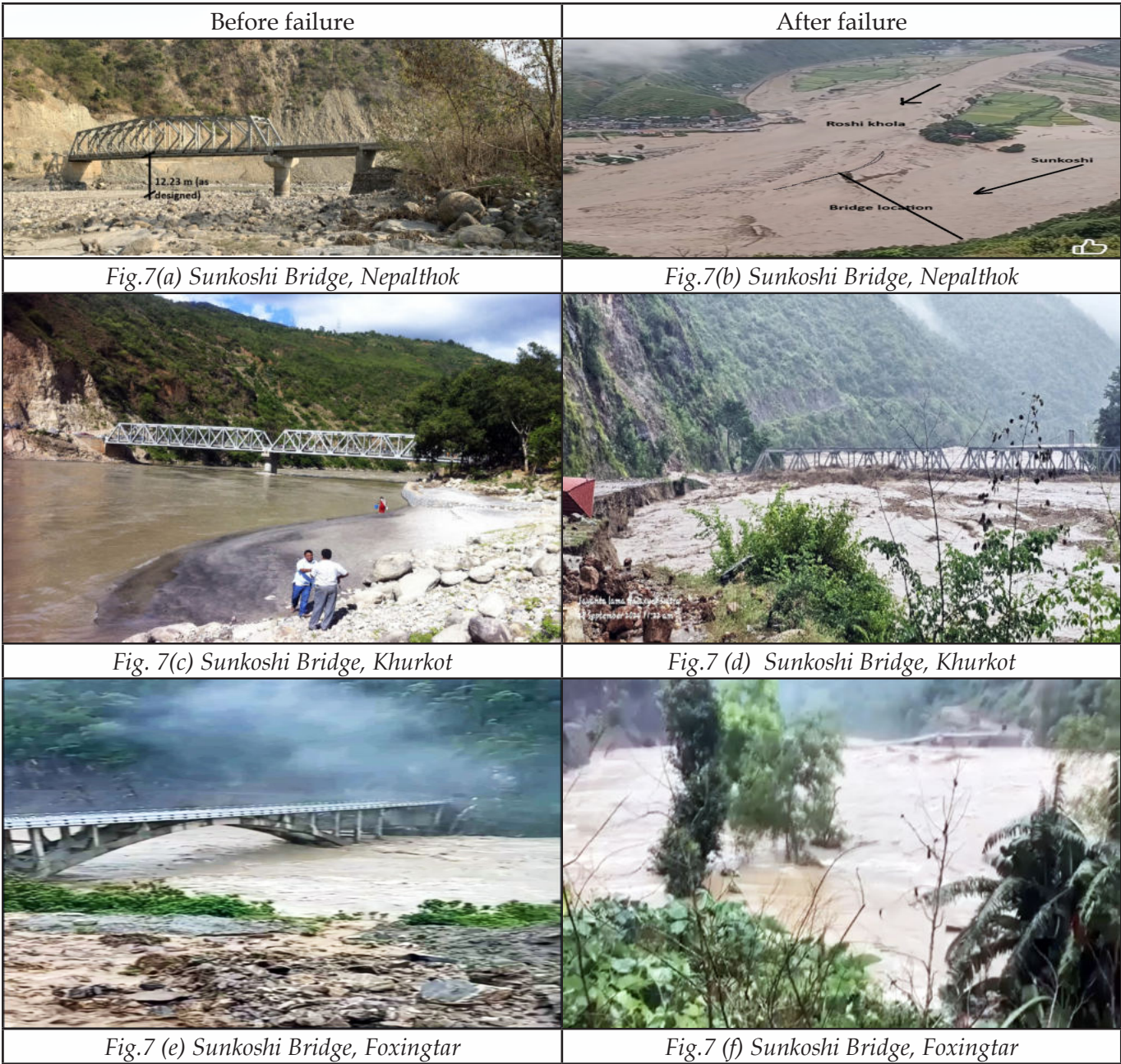
Fig.7 Photographs of various bridges in Koshi Basin before and after failure that are collapsed due to record breaking extreme flooding of 2024/9/27-2024/9/28.
