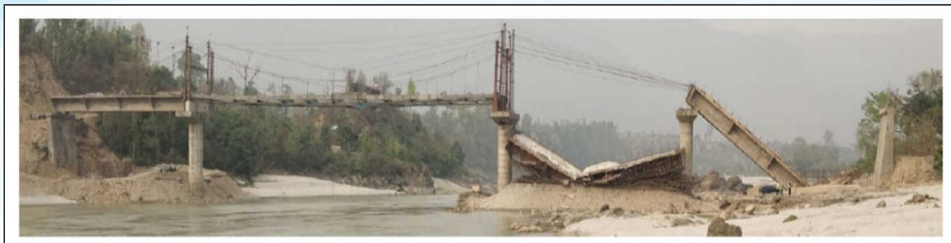
Fig.4(e). Failure of Thimura Bridge during construction ( in 2021-04-06)
