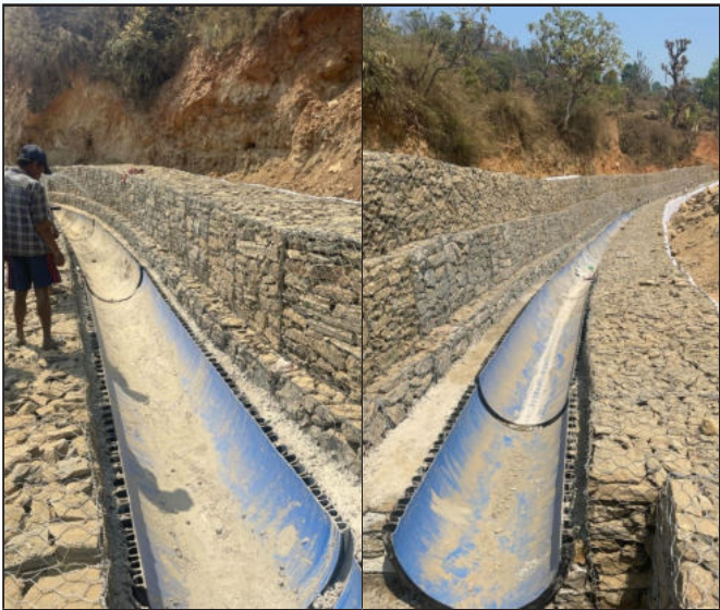
Figure 9: Semi-circular corrugated HDPE pipe on the top of gravel trench for surface drainage.
