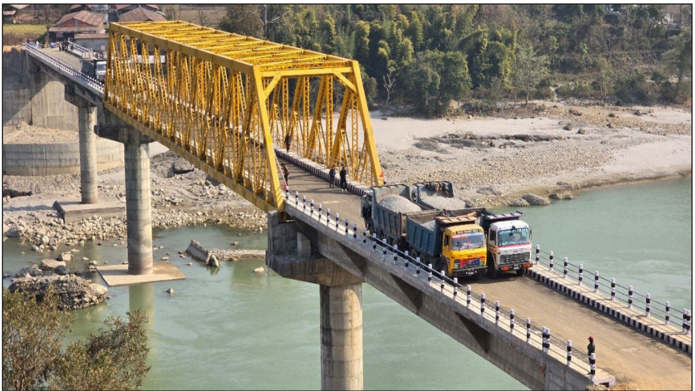
Figure 5: Bridge Load Test on PSC Span and Truss Span
