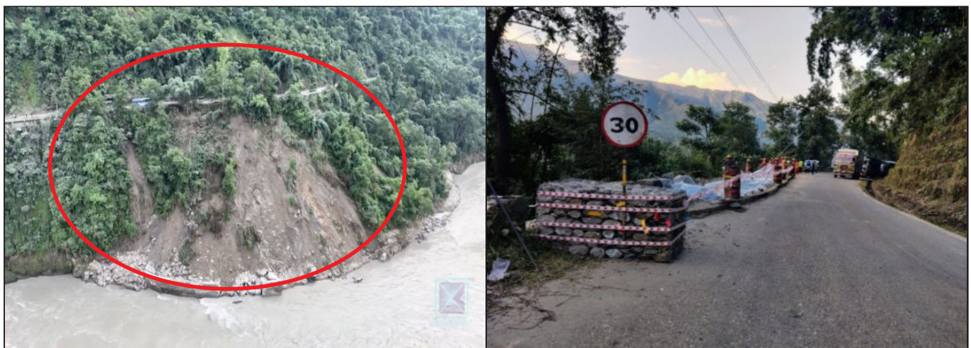
Figure 10: Failure of toe wall and restricted traffic flow at Krishnabhir area.
