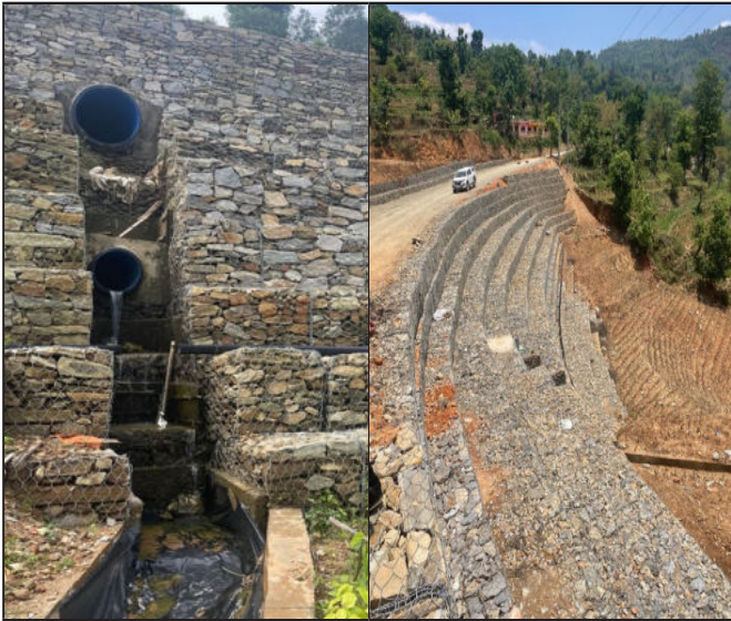
Figure 12: Functioning of sub-surface drainage outlets (left) and completed gabion structure, bioengineering works and drainage chute construction on the right.
