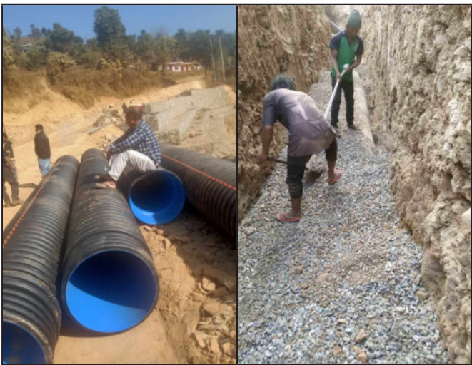
Figure 8: Corrugated half side perforated HDPE pipe
