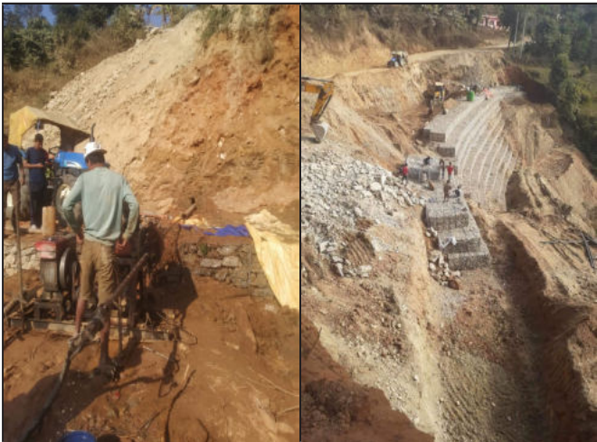
Figure 11: Drilling works for horizontal drainage on left and gabion sleep wall construction on the right.
