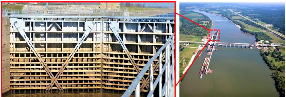
Fig. 1. Greenup locks and miter gate.
