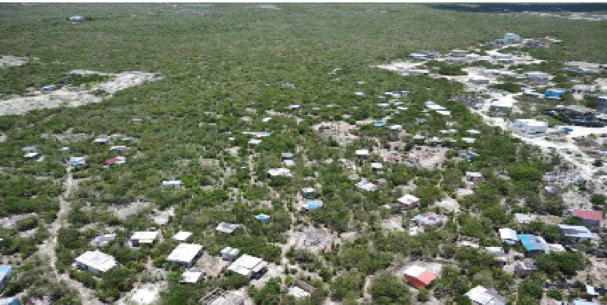
The La Tortue area before the demolition exercise
