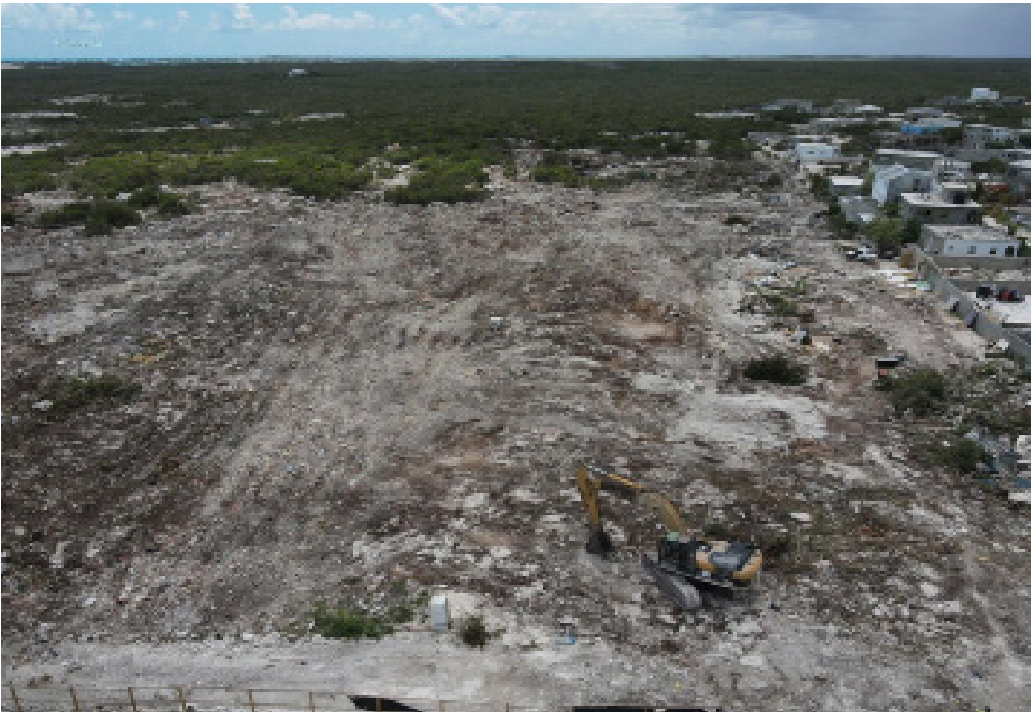
The La. Tortue area after the demolition exercise
