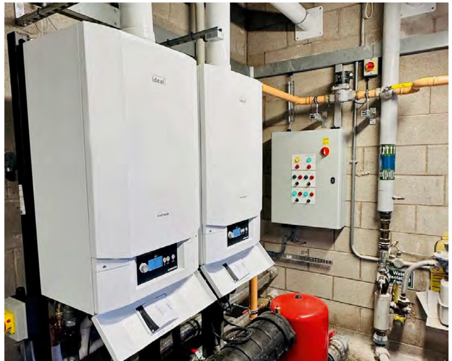
Above: Wall hung commercial condensing boilers at Tinsley Meadows Primary School in Sheffield
