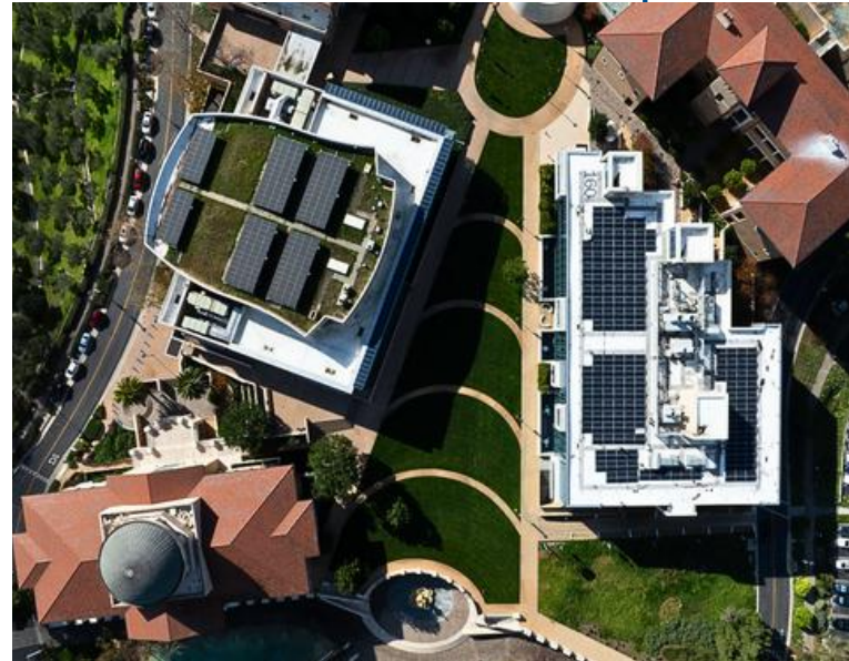
Aerial view of Soka University solar panels and green roof
