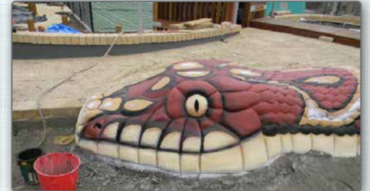
Image 5 - Second Coat of Paint to head
