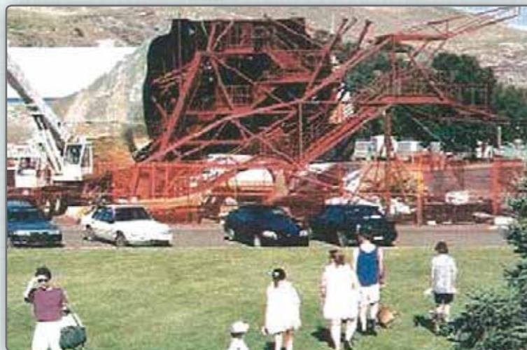
Stage 4 Installation - Inside Steel Armature
