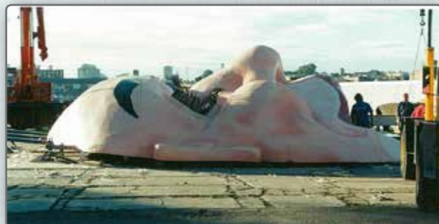
Stage 5 - Delivery - Once the face was delivered it was craned into position and installed on site
