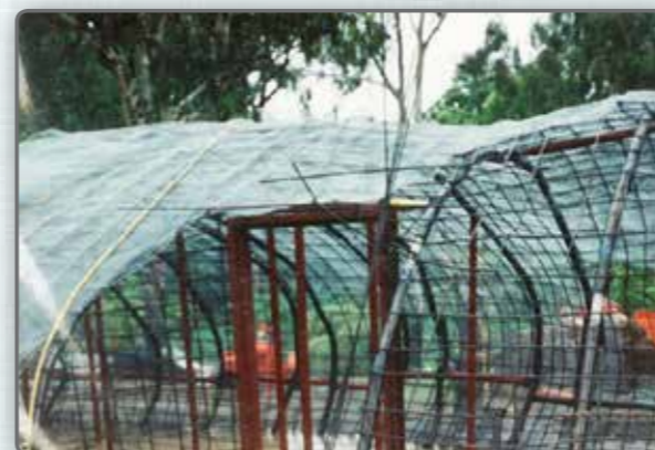
Stage 3 - Adding the door frames & application of wire netting over 10mm mild steel bar armature, which provides the framework for the sturdy concrete finish.
