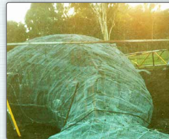
Stage 4 - The steel armature ready to receive the first layer of render
