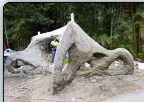
Concrete over mesh
