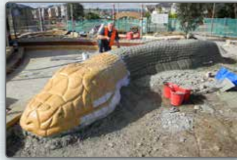
Image 3 - First Coat of Paint being applied
