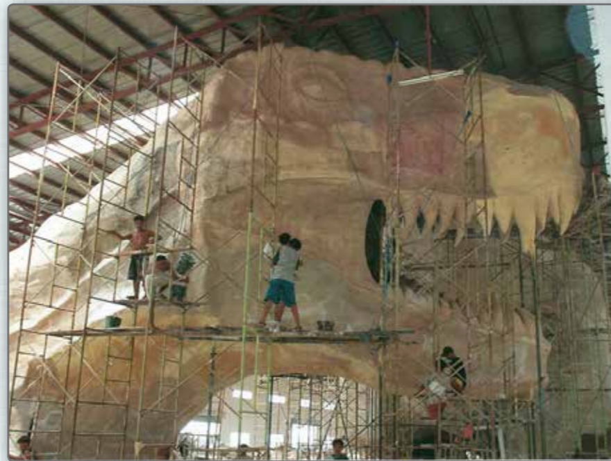
Stage 2 - Scaffolding Around the Head & Neck
