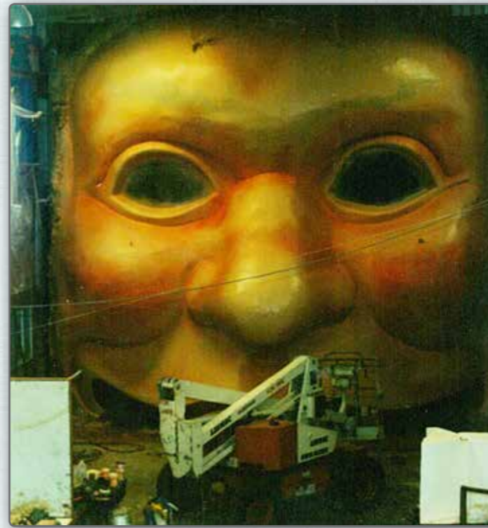
Stage 3 - Once the polystyrene sculpture was perfect, we fibreglassed a heavy duty shell over the front of the piece and then applied a coloured texture to the skin of the face. The styrene became sacrificial.
