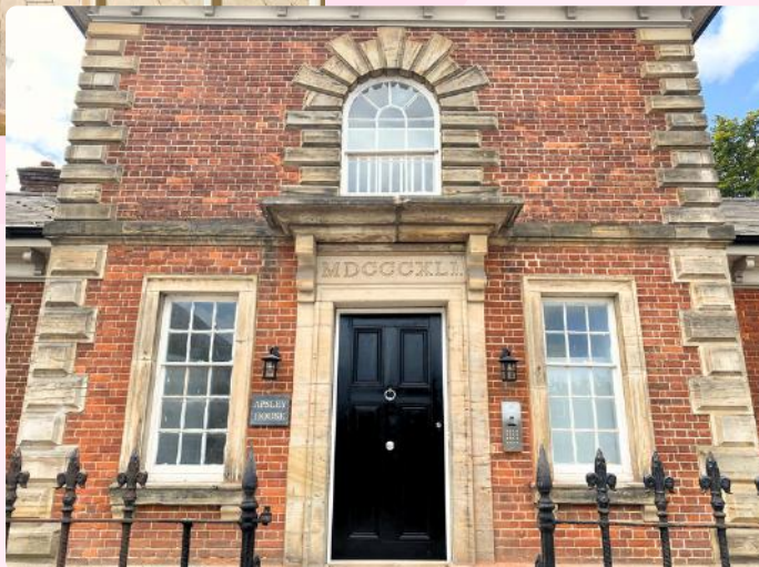
Apsley House Construction and Exterior
