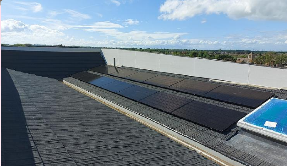
Albany Court Undercroft Construction and Roof
