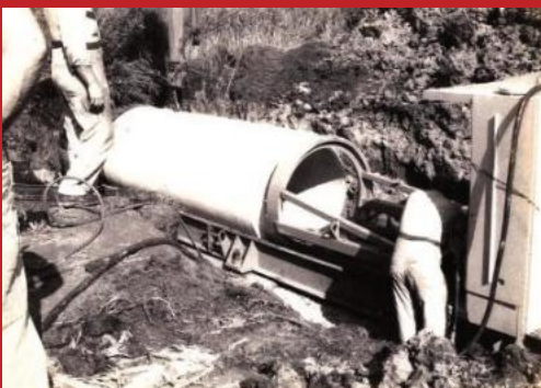
| Akkerman pipe jacking system. Circa 1960's
