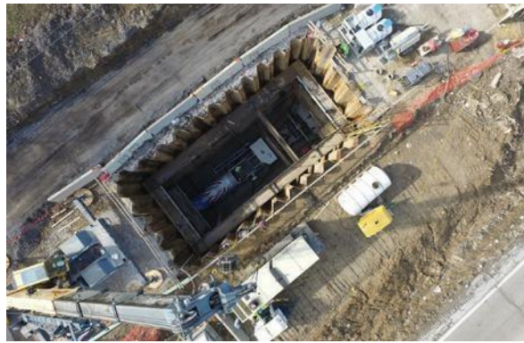
Figure 5: Akkerman pipe jacking system launching from driven sheet pile shaft construction.
