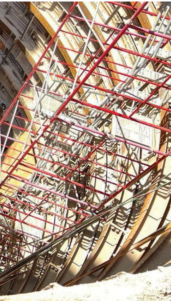
↑ SR-51 Launch shaft setup.
