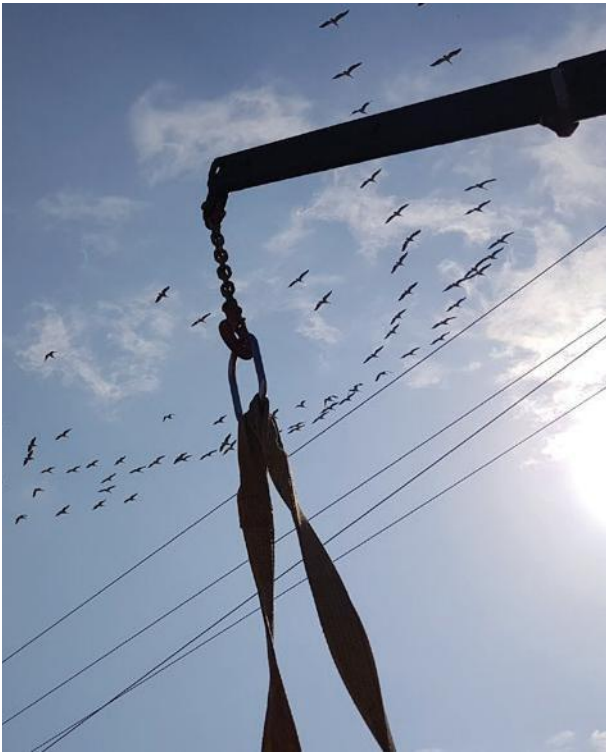
Figure 4: Example of an aerial hazard that could influence jobsite safety and efficiency.
