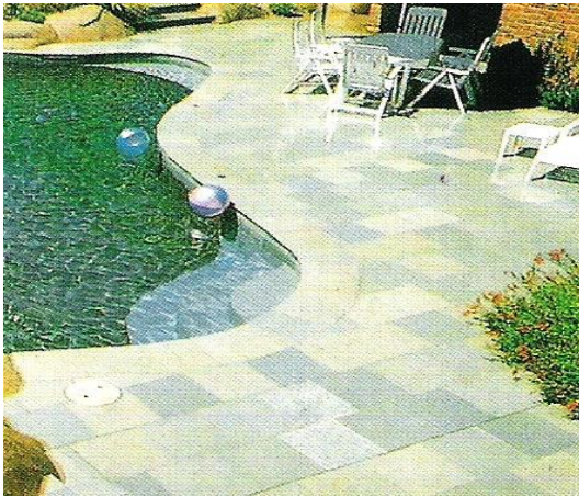
Slates for pool paving
