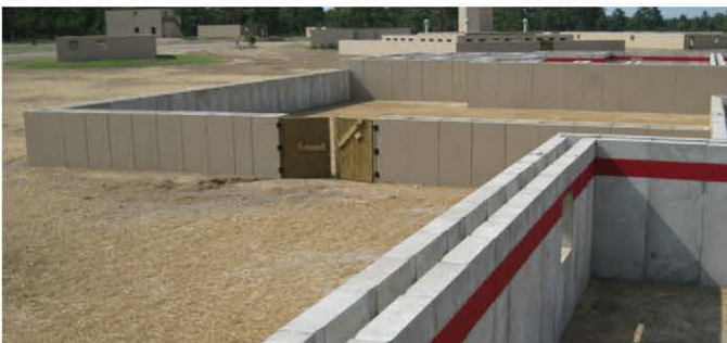
Live-Fire Building MOUT Site
