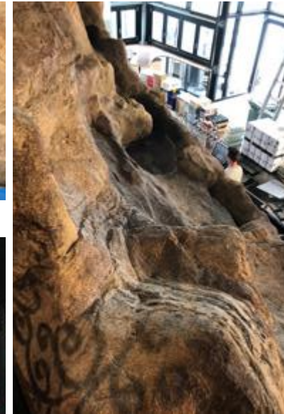
Installing the rock wall and waterfall
