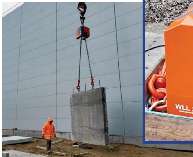
The pewag levo load balancer is suitable when the load has to be lifted horizontally or at a certain angle and is available for hire nationwide.
