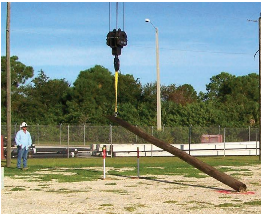
Fig. 2. A vertical sling keeps the pole from sliding.
