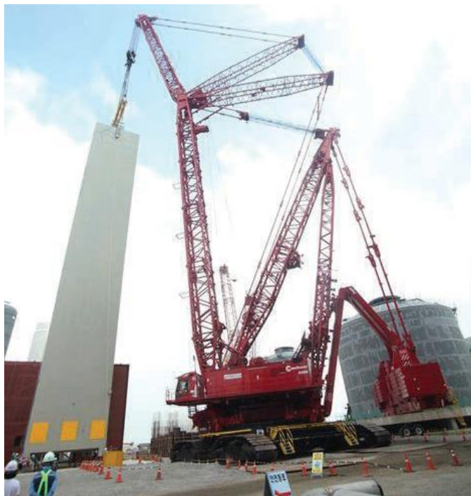
Fig. 1. A 2024 Manitowoc 32000 heavy lift crawler crane.
