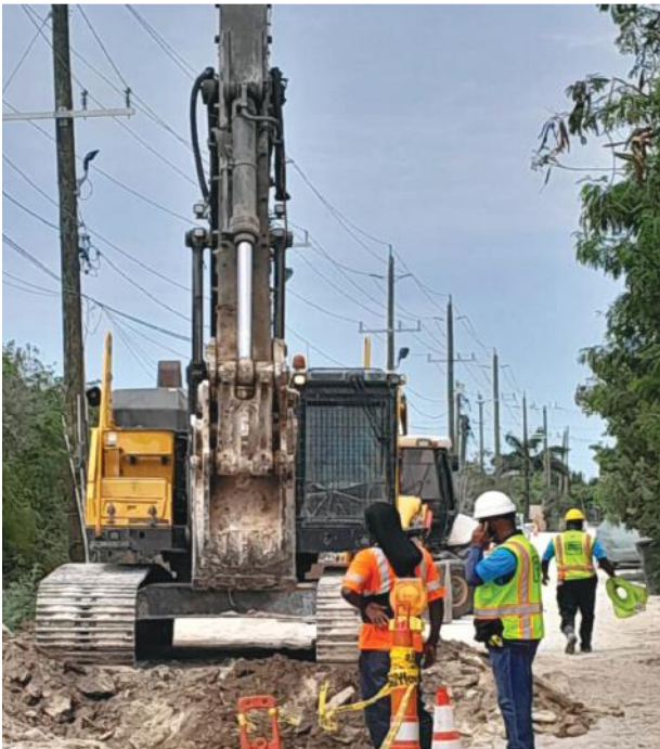
PWC Workmen cutting new trenches to lay pipes for increased water supply
