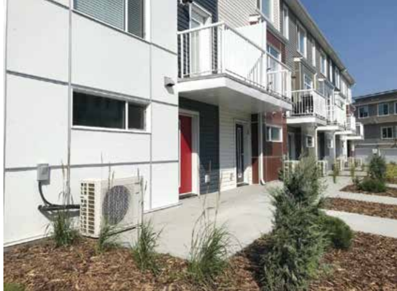
Figure 3. Exterior photo taken at end unit of case study building.
