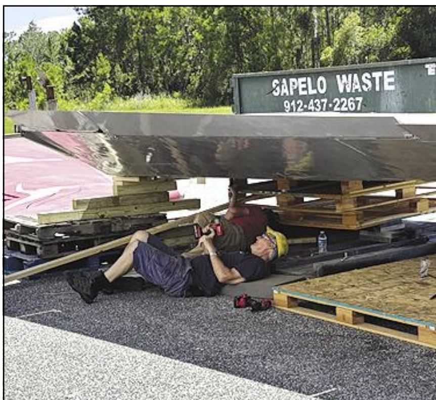
Working under the stabiliser to remove access panels to enable elevators to be removed.
