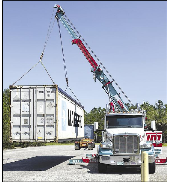
Loading the containers.
