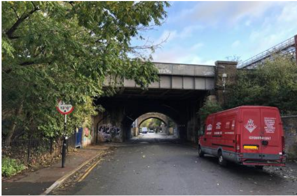
3.2 Reduce carriageway width; increase space for pedestrians and cyclists. Enhanced lighting under the bridge.
