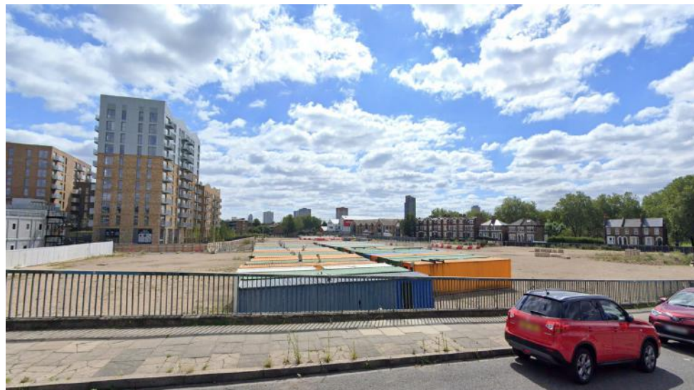
bottom, view of Deptford Landings under construction, from Oxestalls Road bridge.
