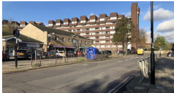
1.6 Grove Street/Longshore Street: environmental improvements to improve crossing, remove unnecessary guardrails, improve rubbish facilities, and add trees and planting.
