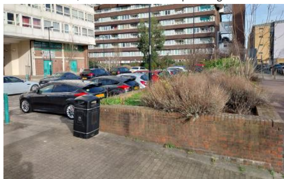
1.9 Greening landscape around Daubenay Tower including restoration of original brick planters.
