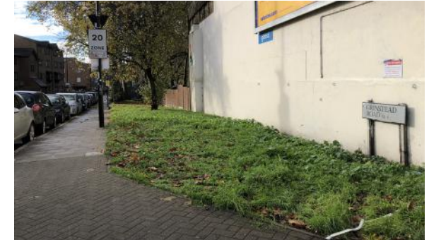
4.2 Opportunities for tree planting and/or rain garden at Evelyn Street/Grinstead Road junction.
