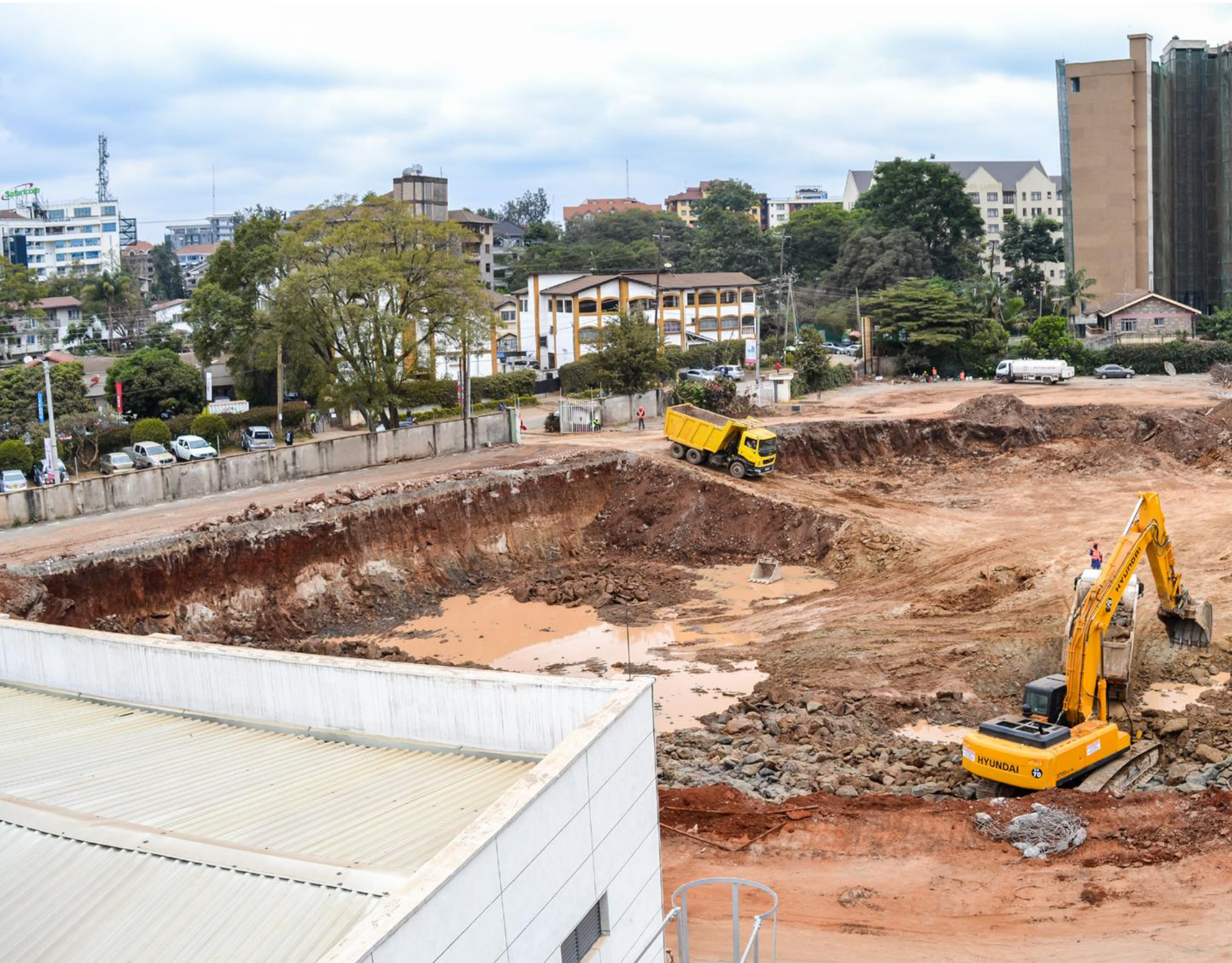
Phase 3 construction site.
