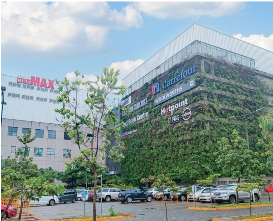
Left: The ten-storey parking lot with 950 parking space and an external natural green wall with a gym, and entertainment area on the top floor.
