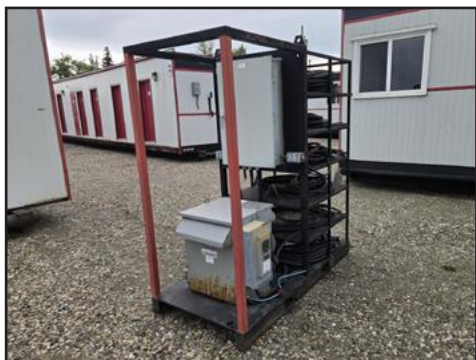
3 Phase 45kVA Transformer On Skid
