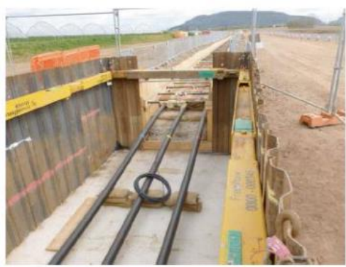
Direct buried cable installation in a rural area
