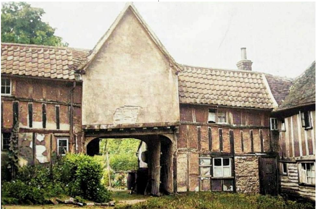
The Courtyard before restoration - 1952
