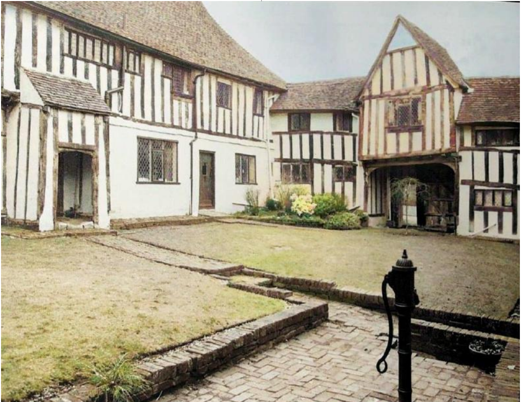
Courtyard after restoration.
