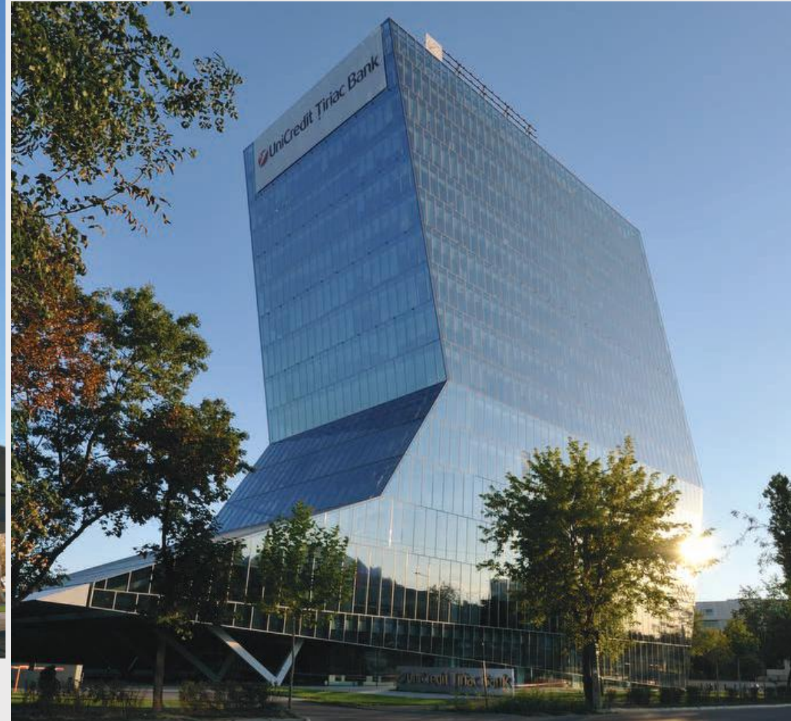
ARACO 2013 Quality Trophy The Special shape of the building required the installation of four seismic dampers
