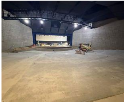
Auditorium: New seats, flooring, lighting and sound, refinishing the stage COMPLETION: SUMMER 2026
