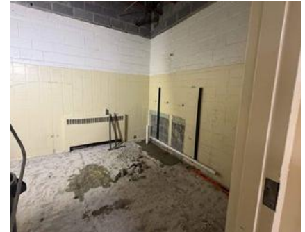
Bathroom Renovations COMPLETION: SUMMER 2026
