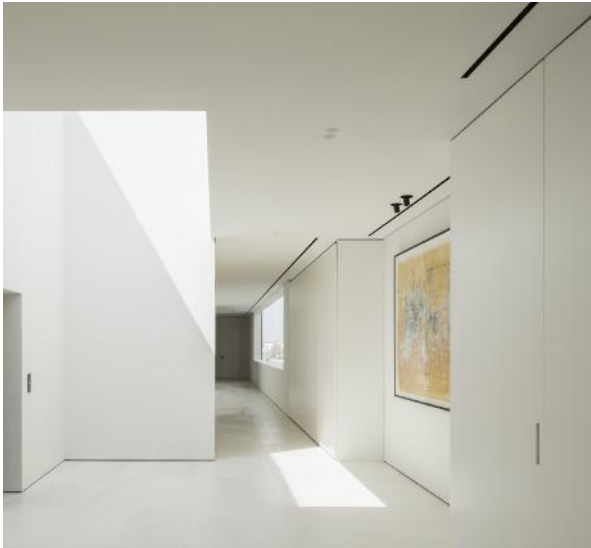
MINIMAL CEILING - LINEAR AC SLOTS
