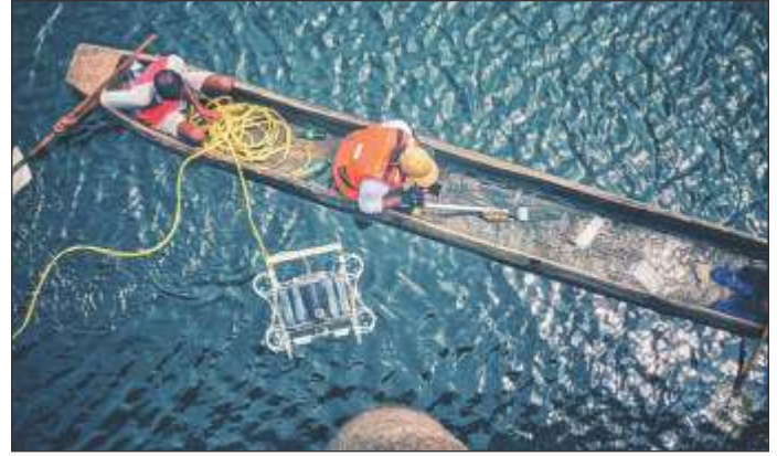
ROVs can capture detailed visual and sensor data that can be stored, analyzed, and compared over time -- enabling predictive maintenance and digital record keeping.
