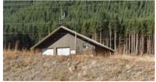
PCFD 25 Station (Google Street View)
