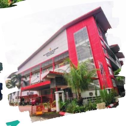
3 HANG TUAH FIRE STATION KL
