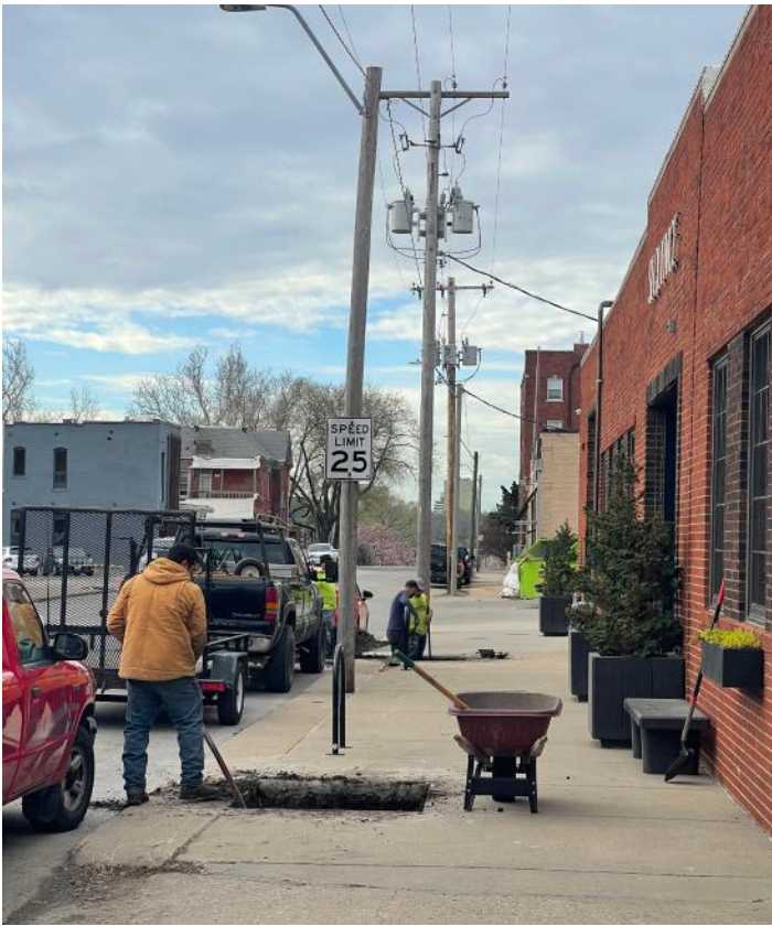
In front of Sequence Rock Climbing Gym, workers put the finishing touches on tree wells that had been jackhammered and excavated. The trees in the newly created wells are Symatree silver maples ( Acer saccharinum ). Photos by Rick Usher
