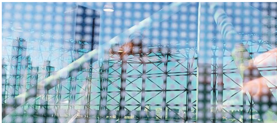
Fritted glass at the Javits Center: In this photo, we see both the reflections of buildings behind the photographer and the New Jersey shoreline through the glass. By making the glass surface itself visible, fritting keeps birds from being deceived by reflections and transparency—and helps them avoid collisions.
