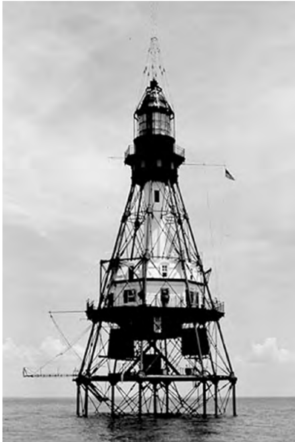
Figure 1.1 Lighthouse supported by screw (helical) pile foundations
