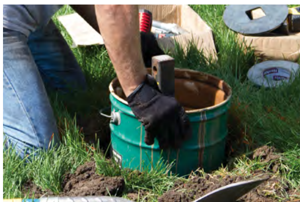
Figure 1.103 Setting the reservoir
