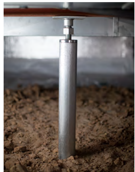
Figure 2.62 Completed concentric pier/SmartJack installation. Model 288 SmartJack shown.
