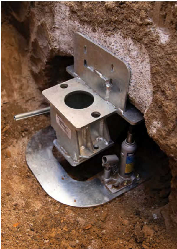
Figure 2.23 Bracket RAYser support system
