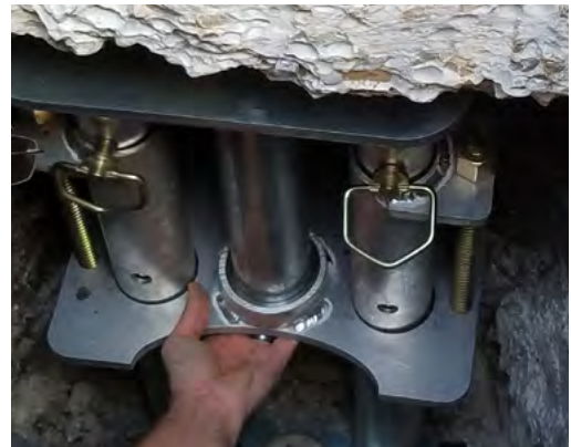
Figure 2.49 Drive stand setup within excavation
