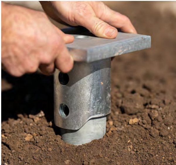
Figure 1.89 Install new construction bracket
