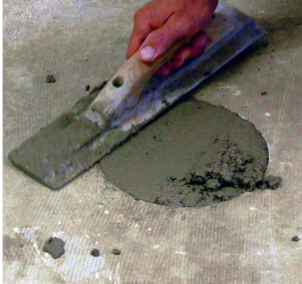
Figure 2.82 Patching holes at pier locations
