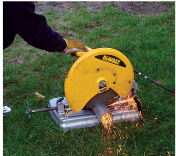
Figure 2.36 Cutting pier tube to desired length with a chop saw
