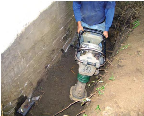
Figure 1.97 Backfill and compact soil
