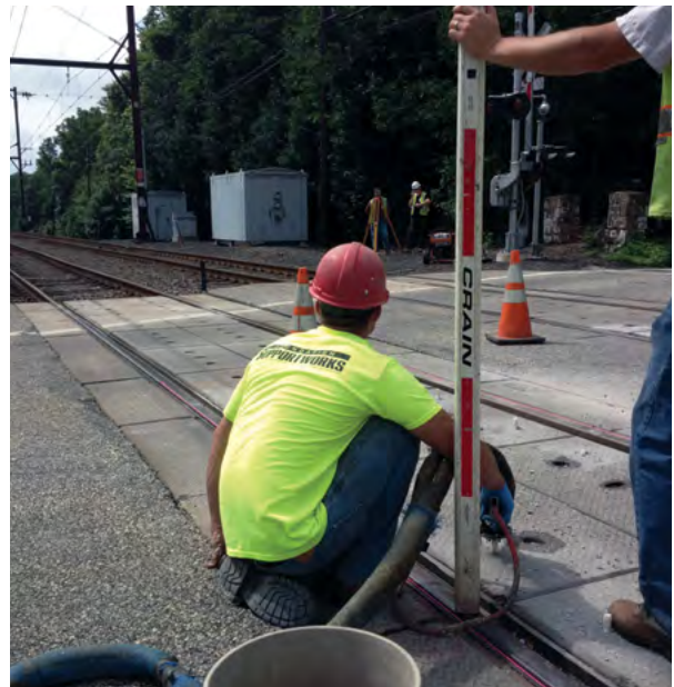
Figure 5.11 Survey equipment used to monitor rail lift from PolyLevel injection
