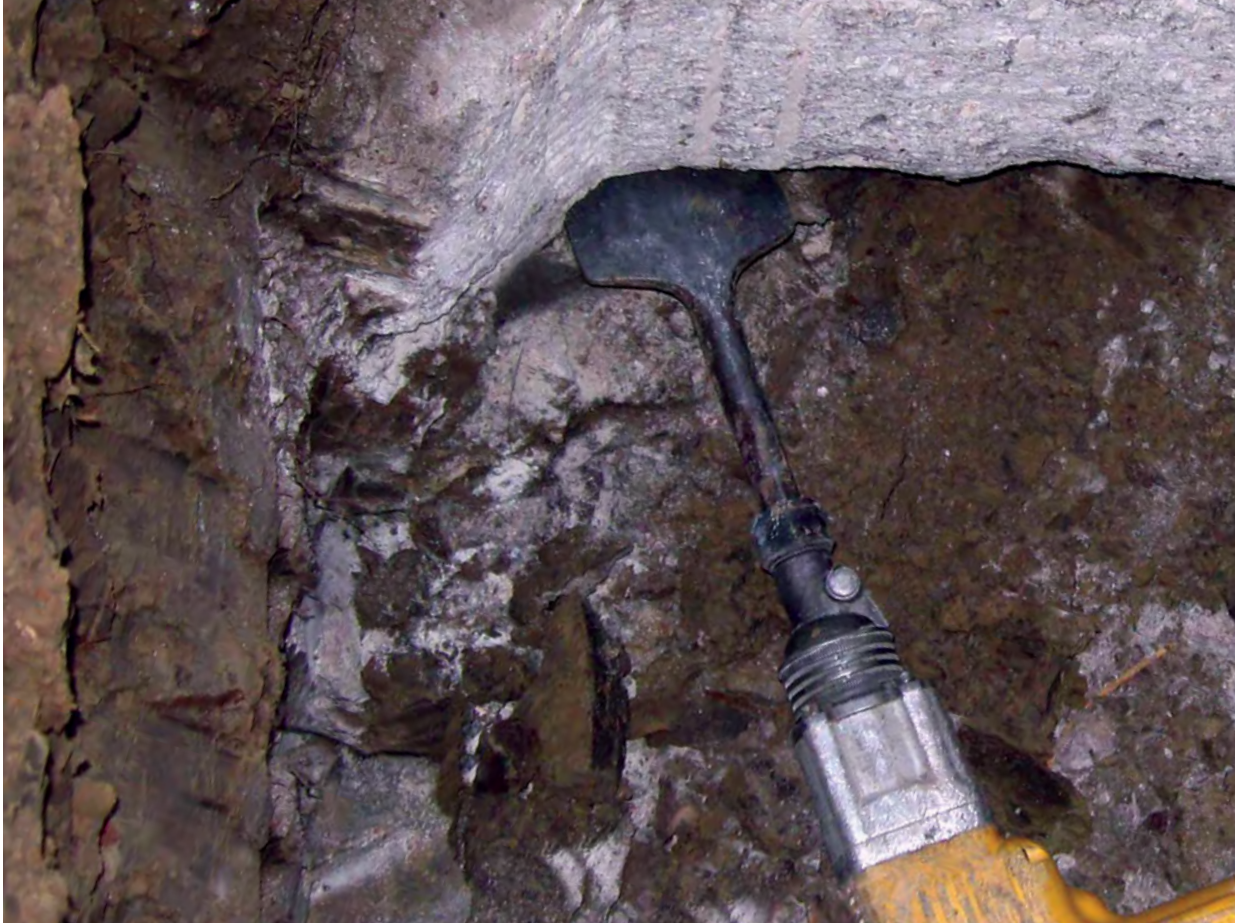
Figure 2.18 Removing soil from beneath the footing with a chisel attachment
