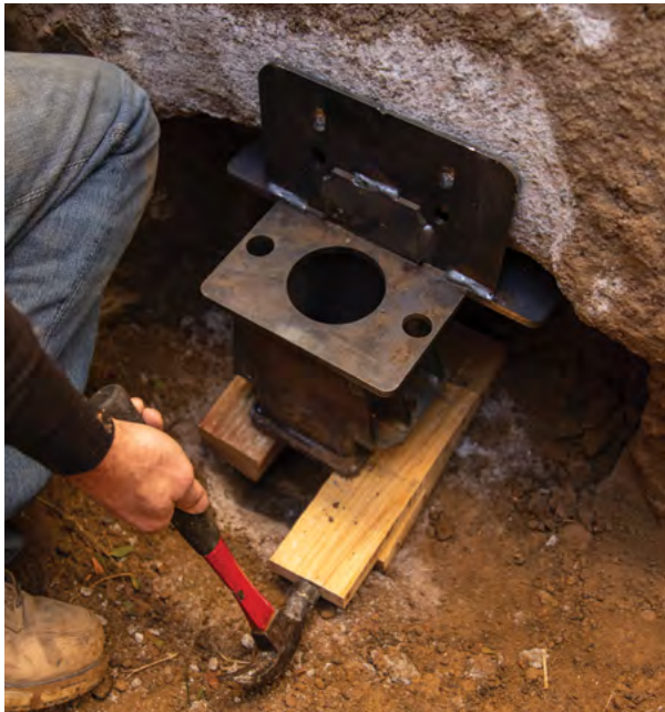
Figure 2.22 Temporary bracket support with wood cribbing
