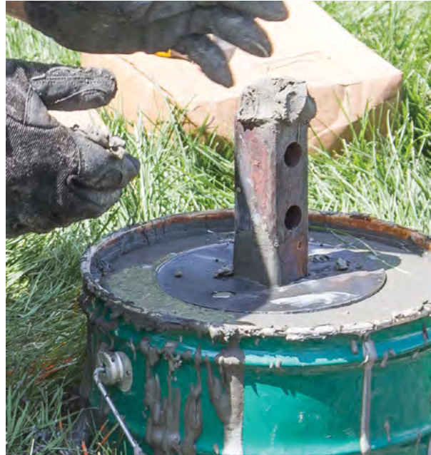
Figure 1.112 Buttering the top of the extension
