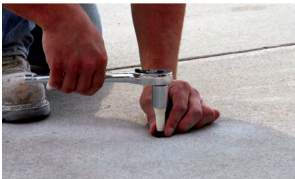
Figure 5.16 Injection port tightened with a socket wrench
