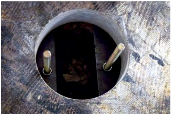
Figure 2.69 Threaded rods installed
