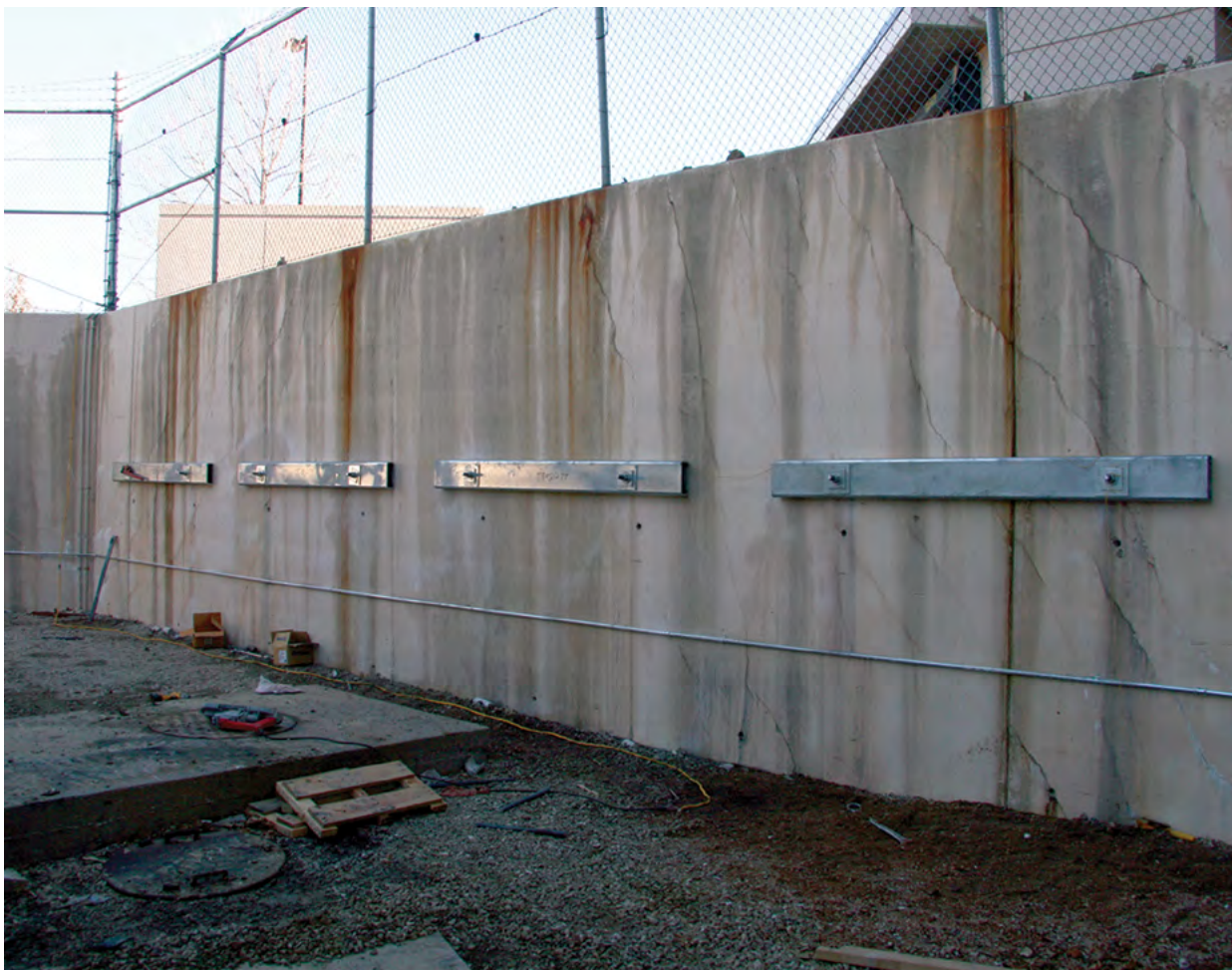
Figure 1.46 Helical tiebacks and tube steel walers stabilize concrete retaining wall
