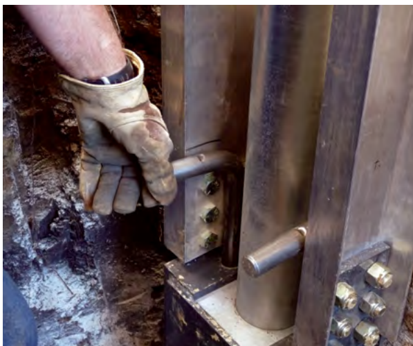
Figure 2.27 PP288 drive stand secured to the bracket with L-pins
