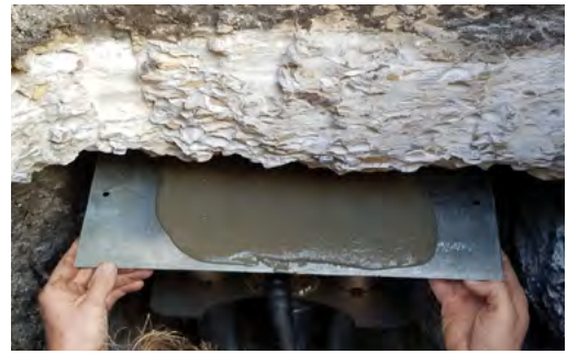
Figure 2.48 Grout plate used to create uniform bearing
