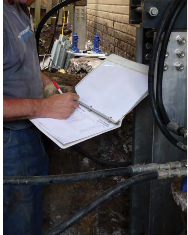
Figure 2.35 Pressure readings are recorded for each pier tube
