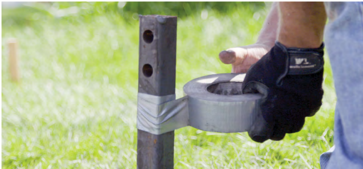
Figure 1.101 Applying duct tape to the lead section
