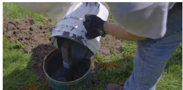
Figure 1.109 Maintaining an adequate level of grout within the reservoir
