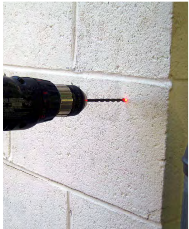
Figure 2.42 Benchmark established with a shallow hole drilled into the concrete block
