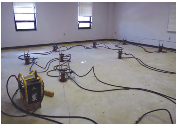
Figure 2.79 Lift cylinders connected for simultaneous loading
