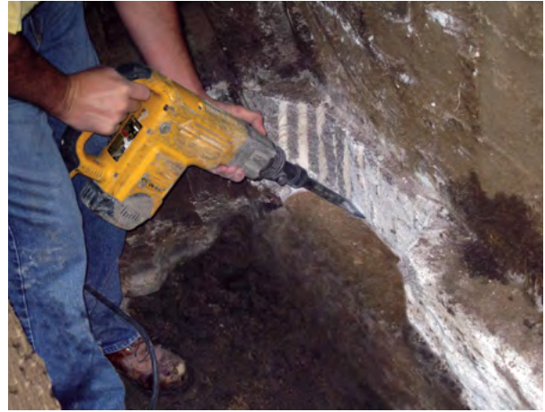
Figure 2.19 Smoothing the vertical and horizontal bearing surfaces with a chipping hammer
