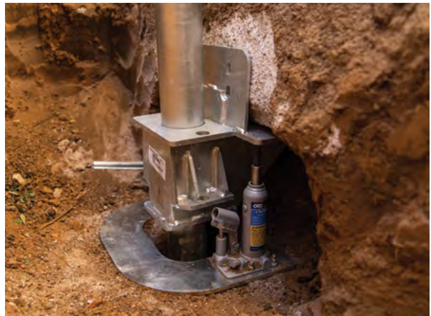
Figure 1.94 Bracket RAYser™
