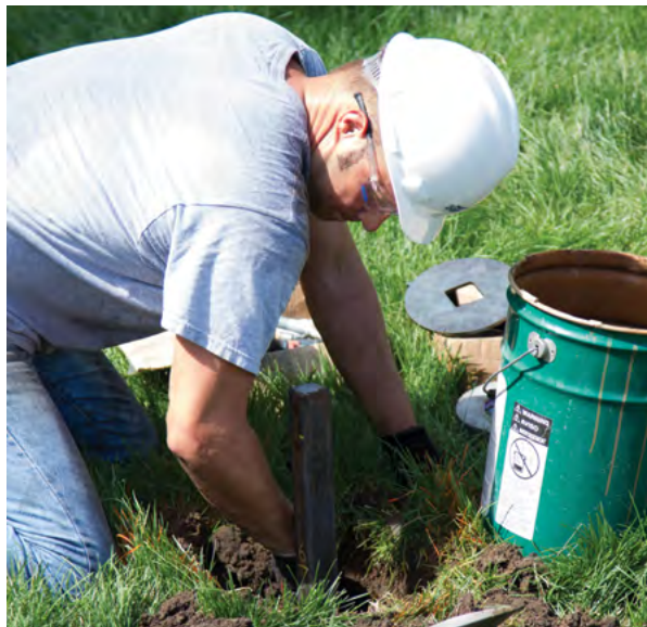
Figure 1.102 Excavating for the reservoir and removing loose soil
