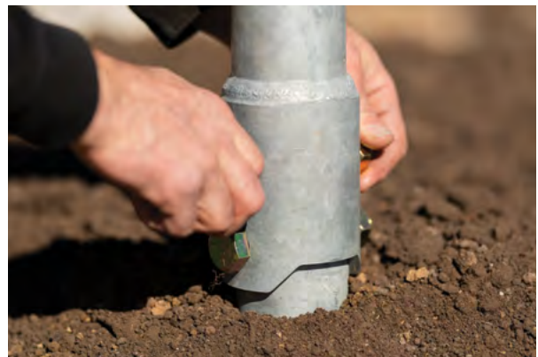
Figure 1.88 Install coupler bolts
