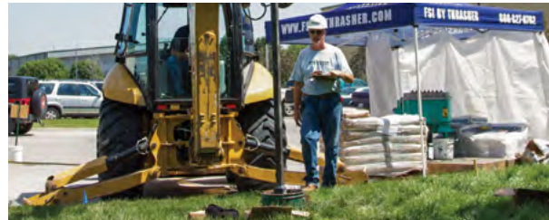
Figure 1.98 Grout mixing station near work area
