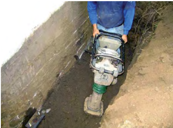
Figure 2.43 Backfill excavations and compact soil
