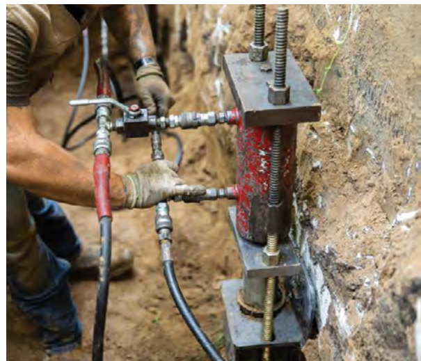
Figure 2.39 Connection of lift cylinder assembly
