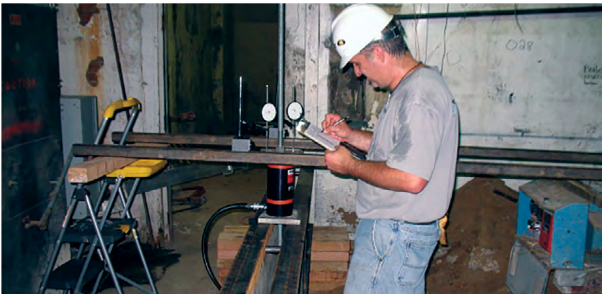
Figure 1.64 Tension load test within basement
