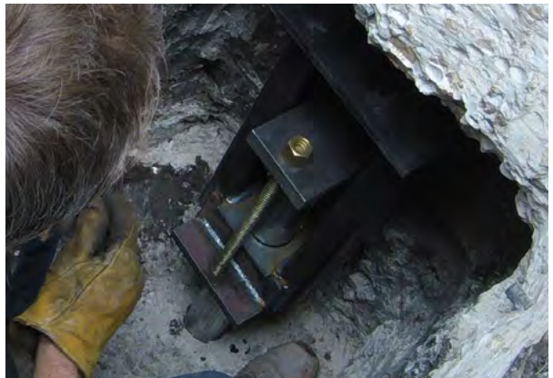
Figure 2.55 Place bracket assembly onto last driven pier tube
