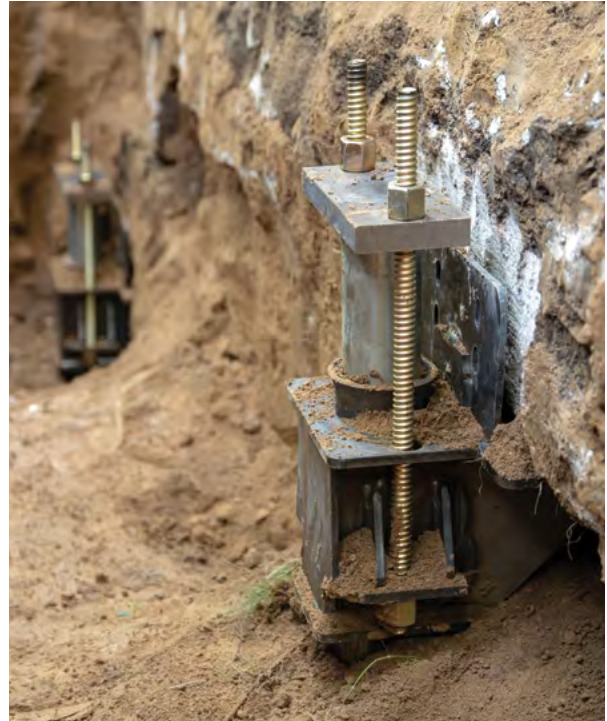
Figure 2.41 System locked off; pier installation complete
