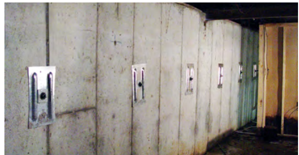
Figure 3.10 After: Wall is immediately returned to original straight position after backfill soil is removed and GeoLock anchors installed
