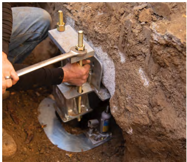
Figure 1.95 Install cap plate and rods
