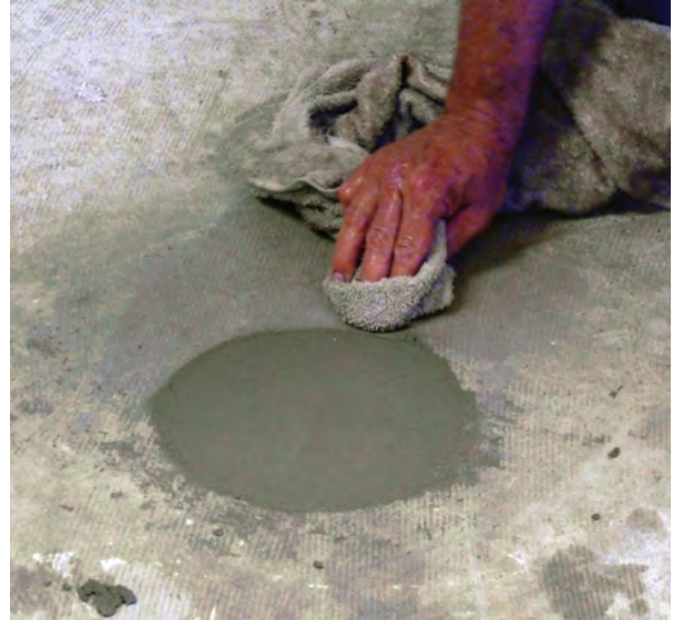
Figure 2.83 Finishing concrete
