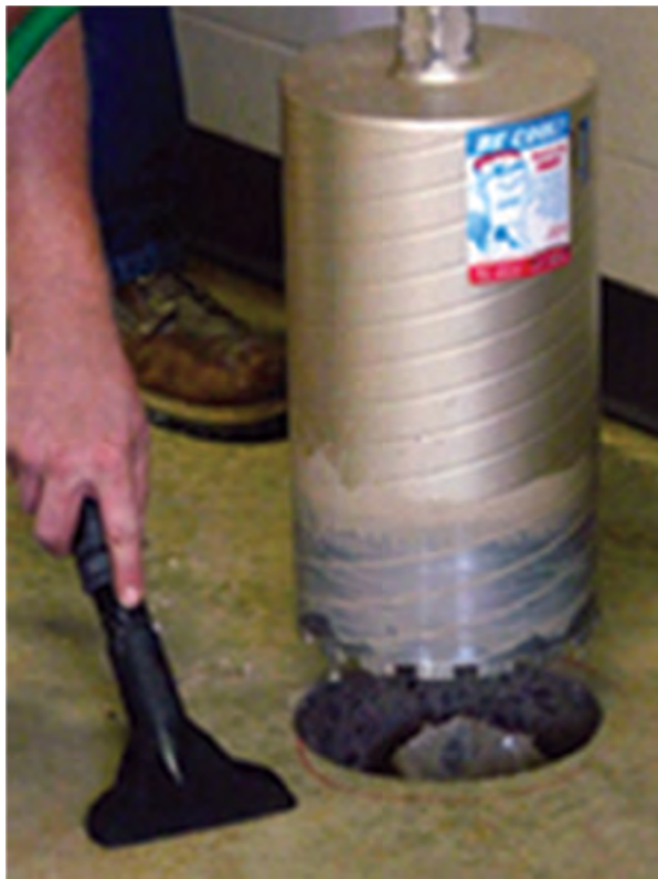
Figure 2.65 Concrete coring
