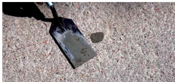
Figure 5.18 Patching the injection hole
