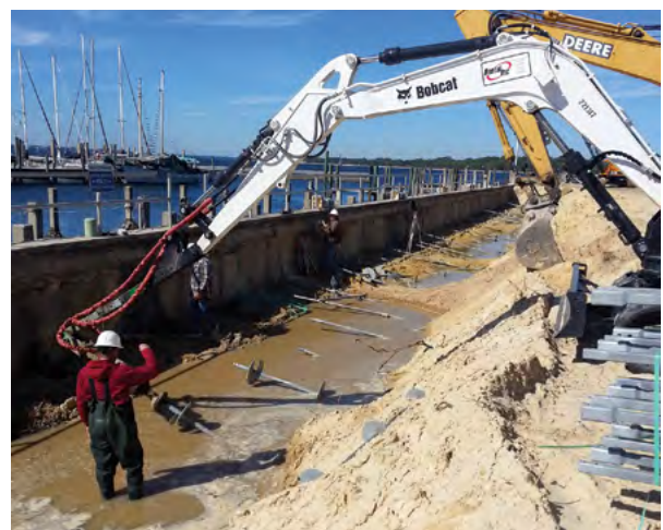
Figure 1.44 Helical tiebacks stabilize marina seawall
