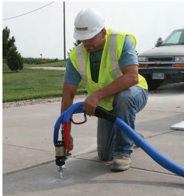
Figure 5.17 PolyLevel foam injected below the slab
