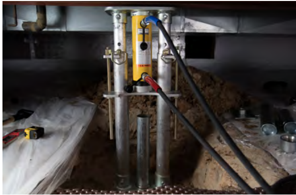
Figure 2.59 Concentric pier drive stand beneath main girder in crawl space
