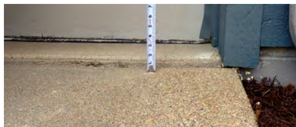
Figure 5.4 After: Driveway lifted back to near original elevation
