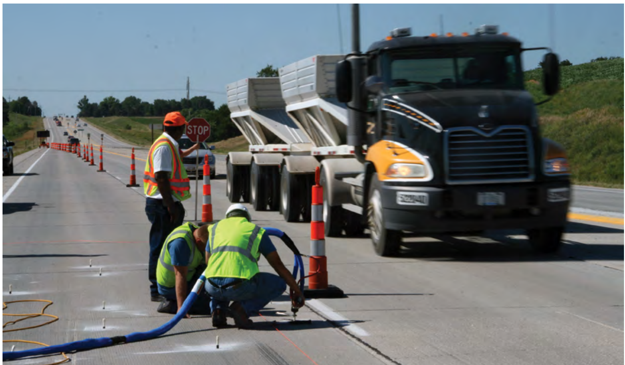
Figure 5.8 PolyLevel injection while maintaining an open lane for traffic
