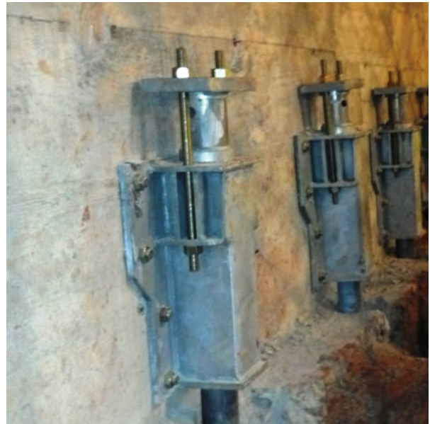
Figure 2.45 Flush-mount bracket installation
