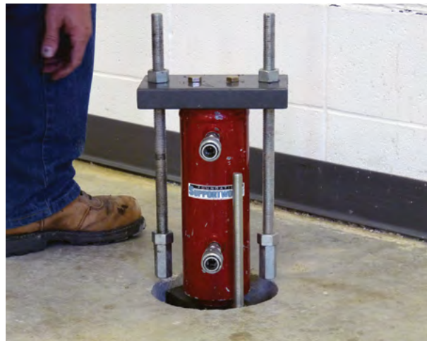
Figure 2.76 Lift cylinder assembly set on pier cap
