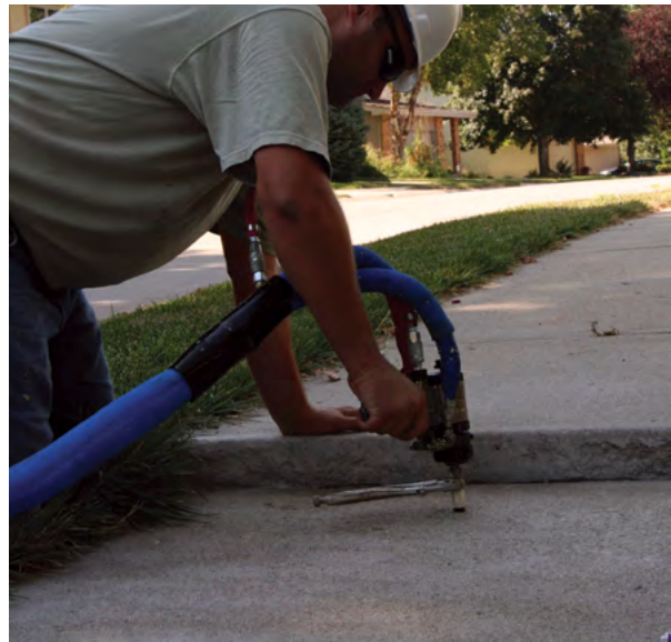
Figure 5.2 PolyLevel foam injected to relevel faulted sidewalk sections
