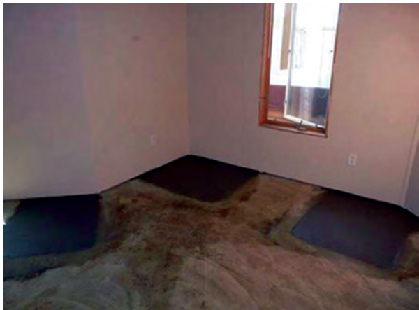
Figure 2.44 Concrete placement at interior pier locations
