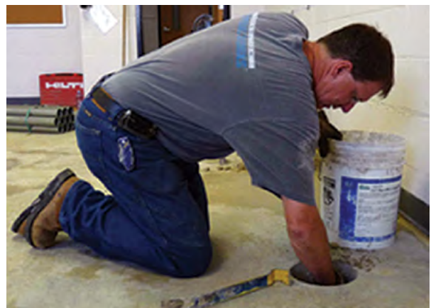
Figure 2.67 Excavating beneath the slab
