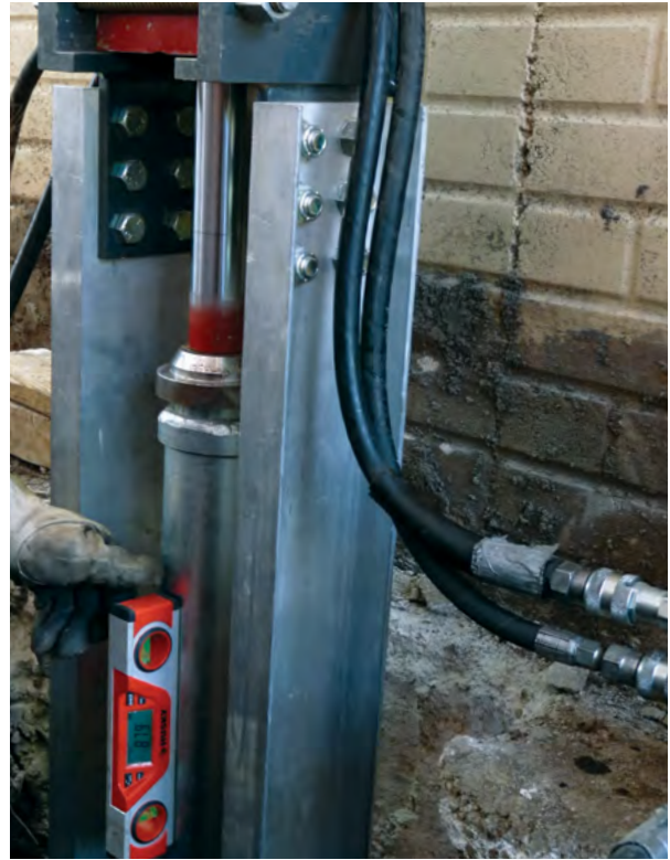
Figure 2.31 Checking drive stand alignment with digital level
