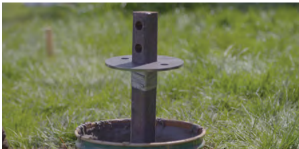
Figure 1.111 Extension displacement plate on the extension shaft
