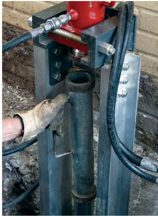
Figure 2.34 Driving tube tool set in place for second stage of push
