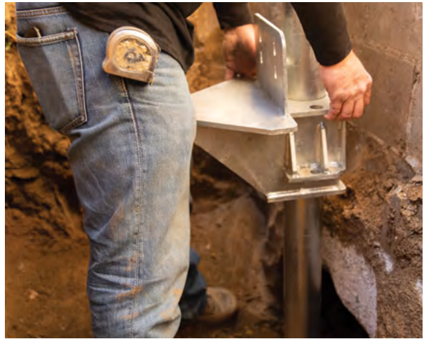
Figure 1.93 Lower assembly over pile shaft
