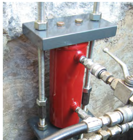
Figure 2.12 Foundation Supportworks FS35LCA lift cylinder assembly
