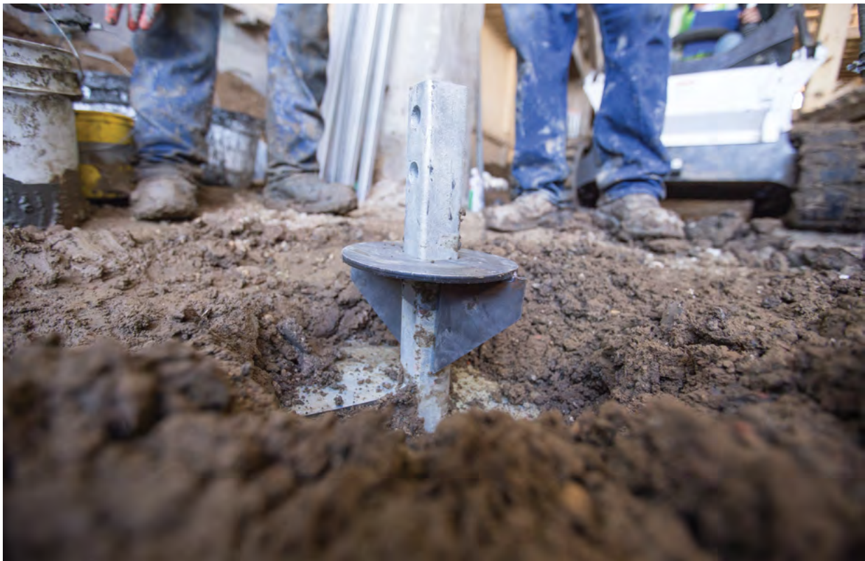
Figure 1.60 Spiked Lead Displacement Plate
