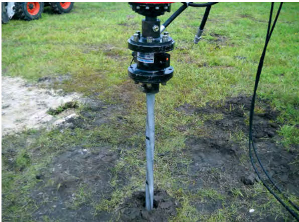
Figure 1.85 Shaft twist
