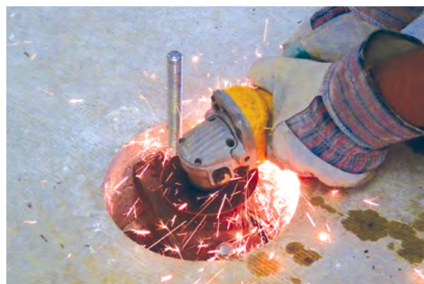
Figure 2.81 Cutting the threaded rods
