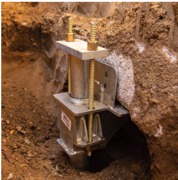
Figure 2.38 PP288 bracket ready for lift cylinder assembly
