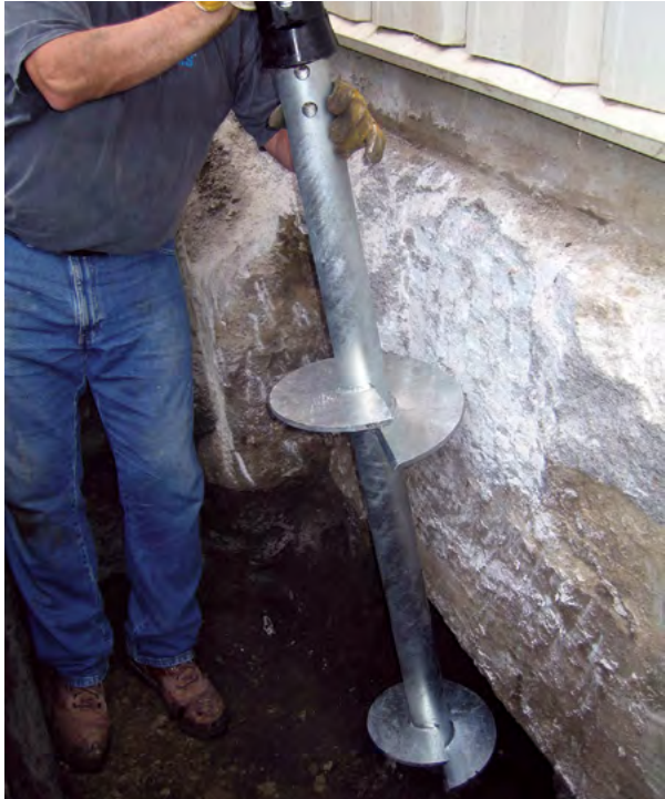
Figure 1.92 Alignment of lead
