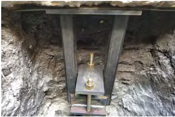
Figure 2.57 Completed concentric pier installation
