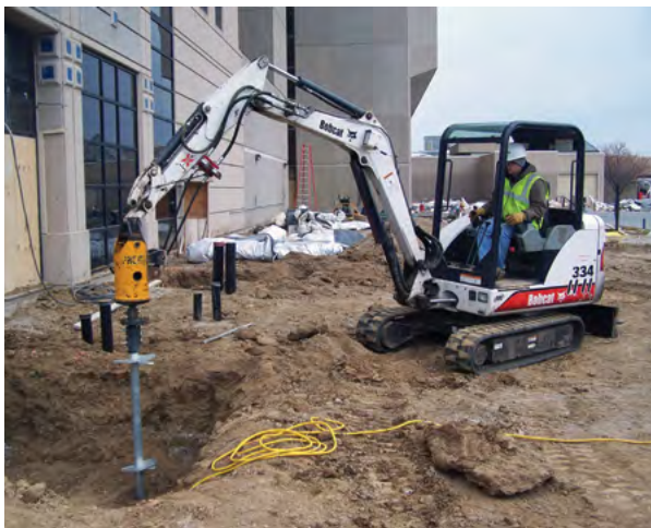
Figure 1.3 New construction helical pile installation
