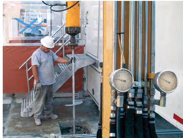
Figure 1.82 Monitoring pressure gauges while installing square shaft helical anchor
