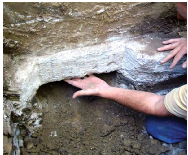
Figure 2.20 Checking underside of footing for proper preparation
