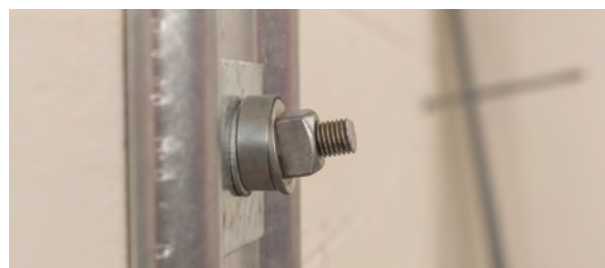
Figure 3.16 Hemispherical washer
