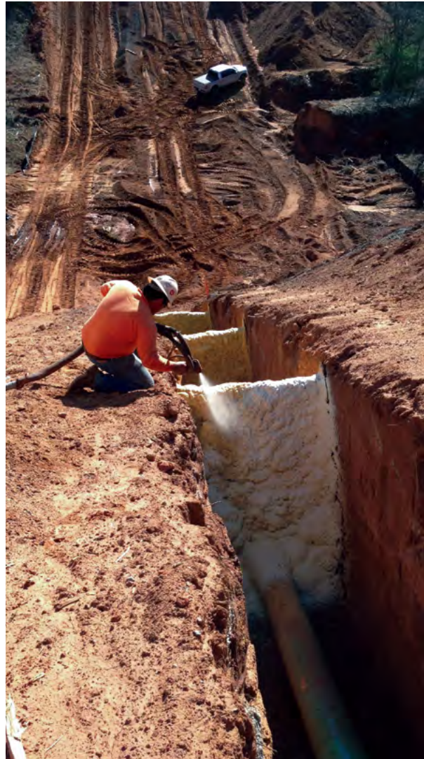
Figure 5.10 Placement of polyurethane foam trench breaks
