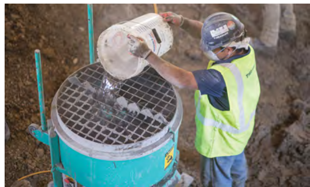
Figure 1.99 Grout mixing
