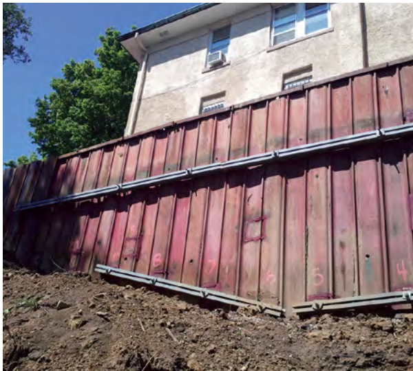
Figure 1.45 Helical tiebacks stabilize sheet pile wall below historic home
