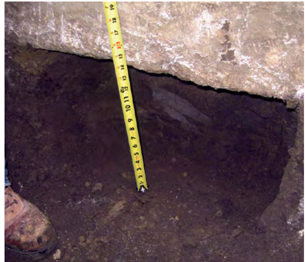
Figure 1.90 Excavation at bracket
