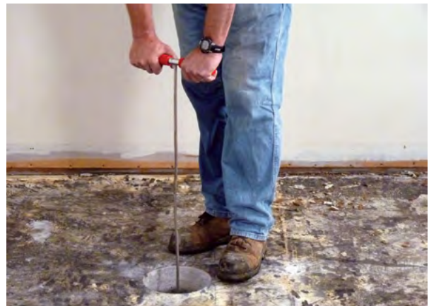
Figure 2.66 Probing for utilities or obstructions
