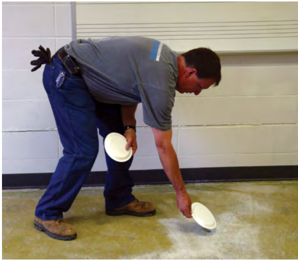
Figure 2.63 Marking slab pier locations
