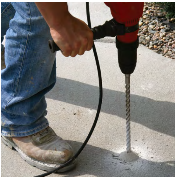
Figure 5.15 Concrete slab drilled to provide access holes
