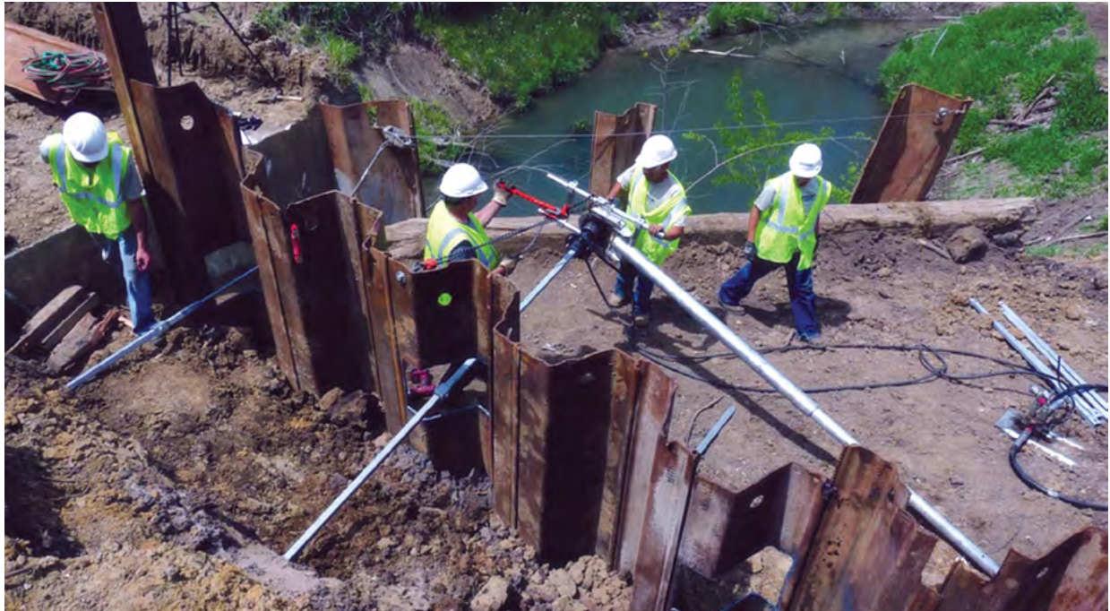
Figure 1.5 Helical tieback installation with hand-held equipment
