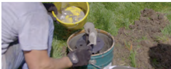
Figure 1.107 Buttering the top of pile at coupler
