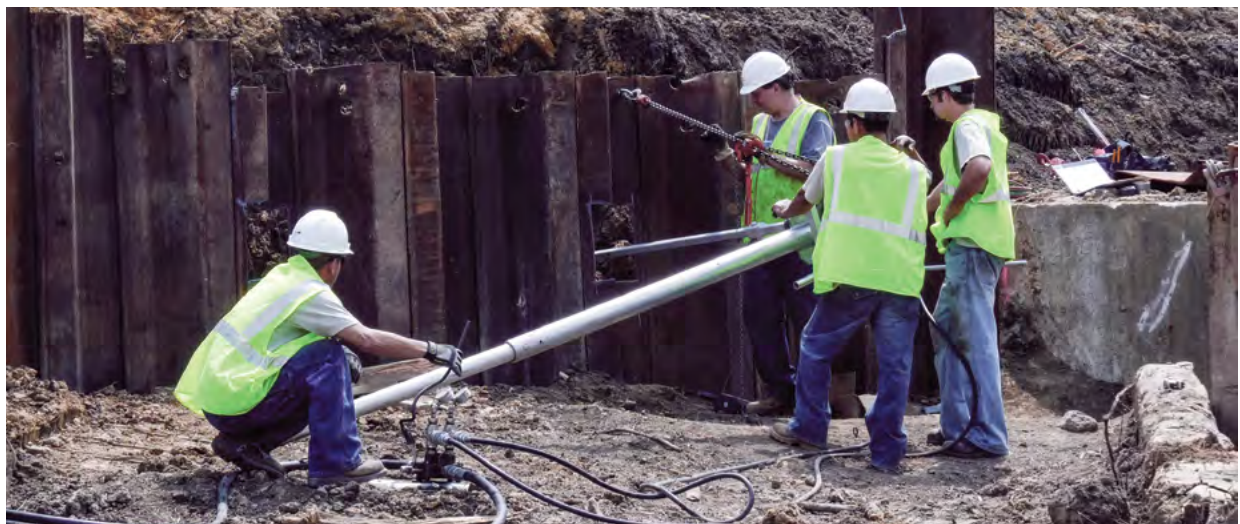
Figure 1.77 Torque arm
