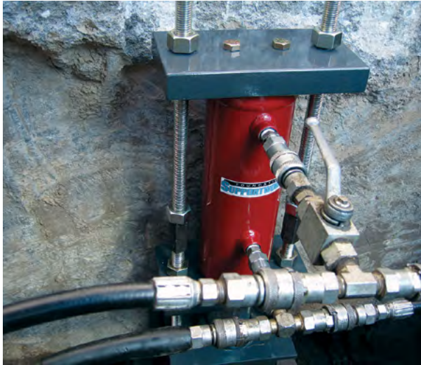
Figure 1.96 Set hydraulic lift cylinders
