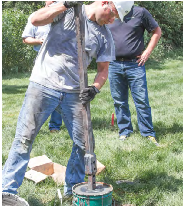
Figure 1.113 Placing an additional extension
