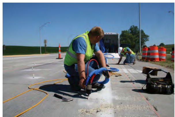
Figure 5.12 Monitoring pavement lift with string lines
