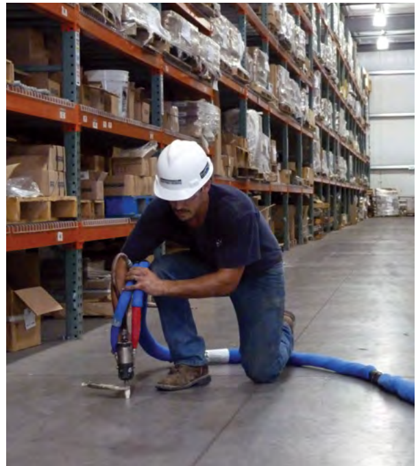
Figure 5.6 PolyLevel stabilizes warehouse floor slab
