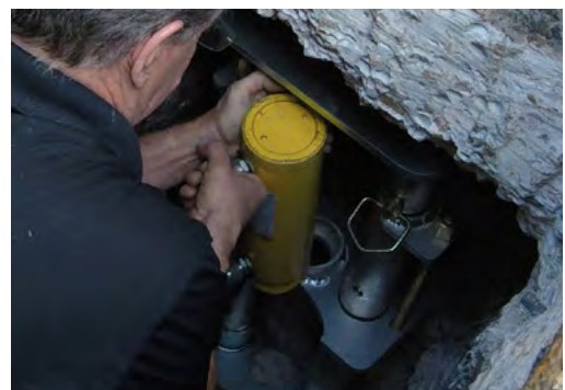
Figure 2.50 Placement of hydraulic drive cylinder
