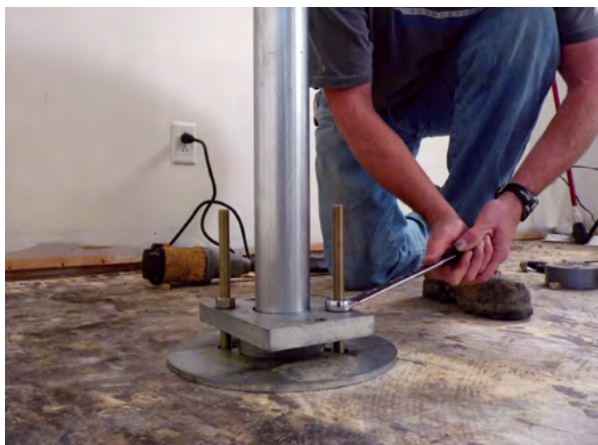
Figure 2.71 Slab pier drive adaptor installed
