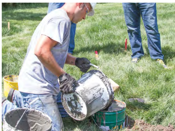
Figure 1.104 Pouring grout into the reservoir
