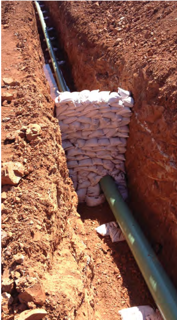
Figure 5.9 Sandbag trench breaker for pipeline
