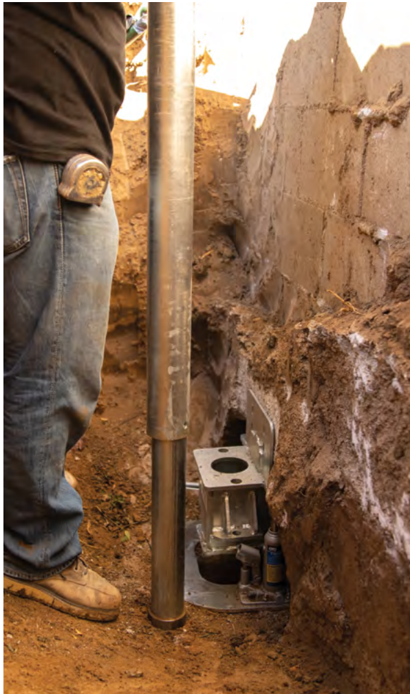
Figure 2.24 Exterior sleeve slid over the starter tube
