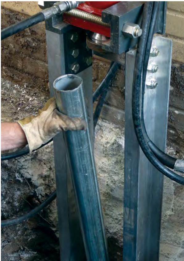
Figure 2.33 Installing PP288 push pier tube
