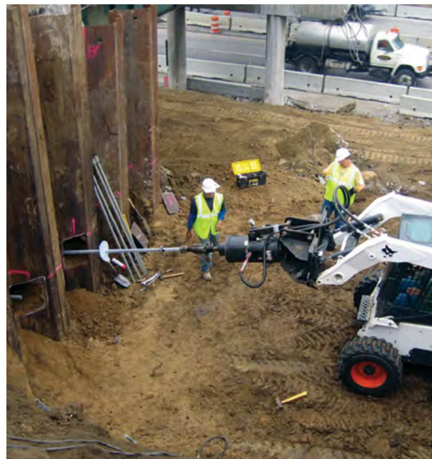
Figure 1.4 Sheet-pile wall stabilization with helical tiebacks
