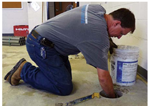
Figure 2.67 Excavating beneath the slab
