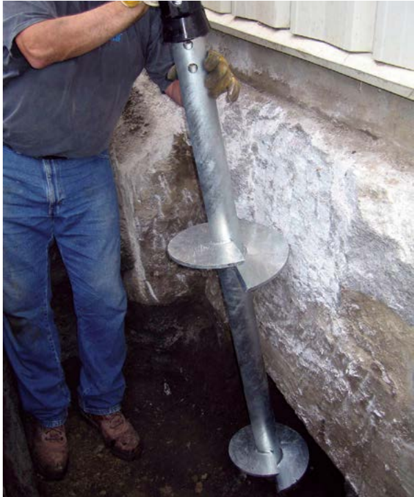
Figure 1.92 Alignment of lead
