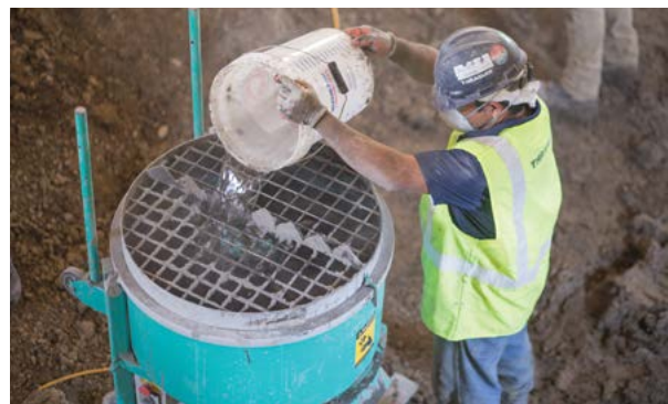
Figure 1.99 Grout mixing
