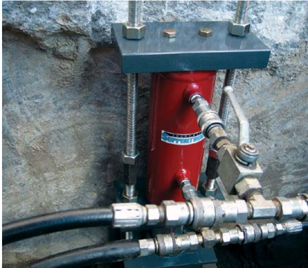
Figure 1.96 Set hydraulic lift cylinders
