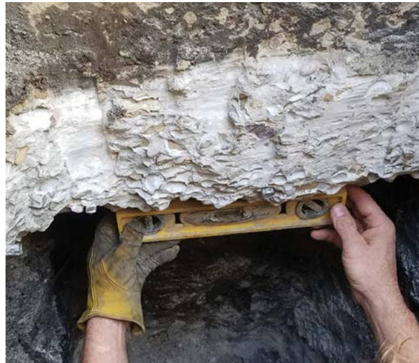
Figure 2.47 Prepare bottom of footing with chipping hammer, as necessary, to create a flat and level surface
