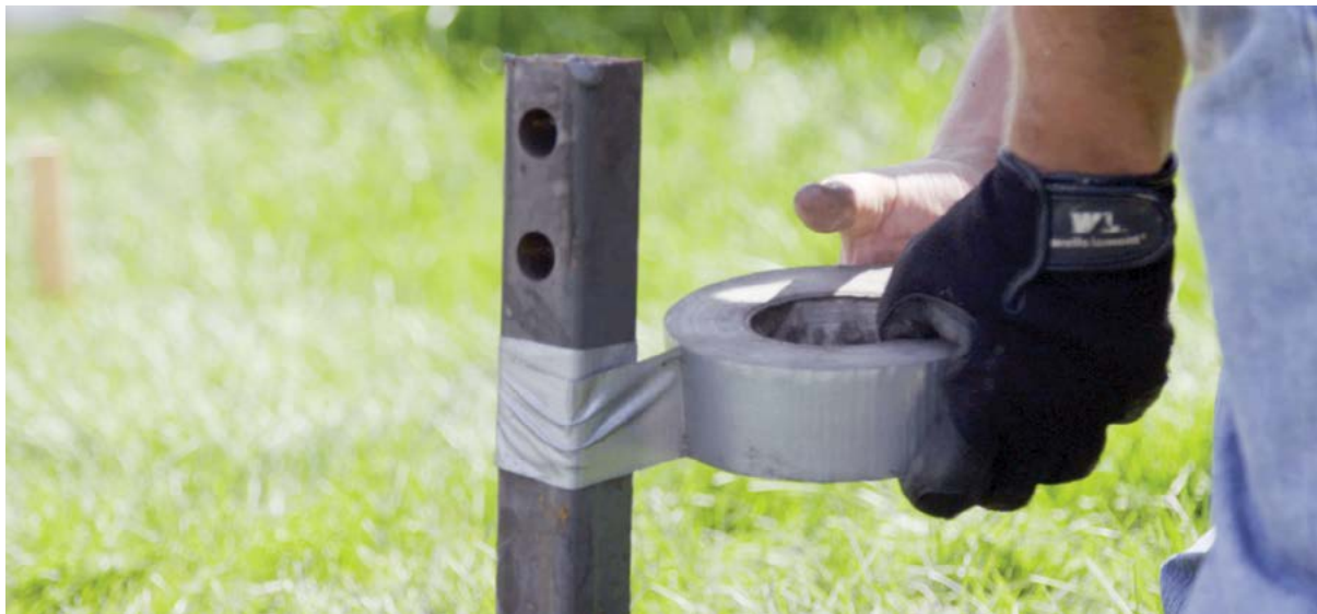
Figure 1.101 Applying duct tape to the lead section
