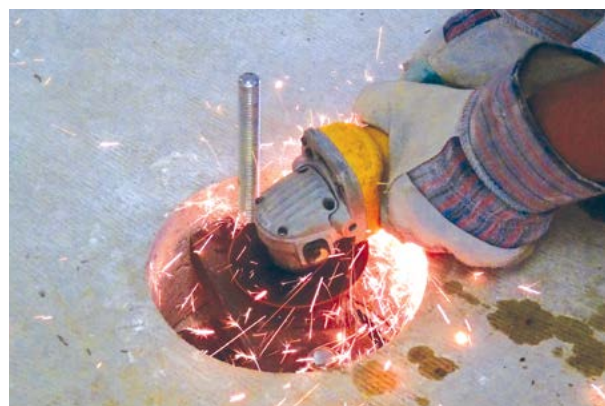
Figure 2.81 Cutting the threaded rods
