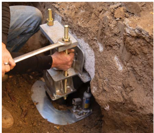
Figure 1.95 Install cap plate and rods
