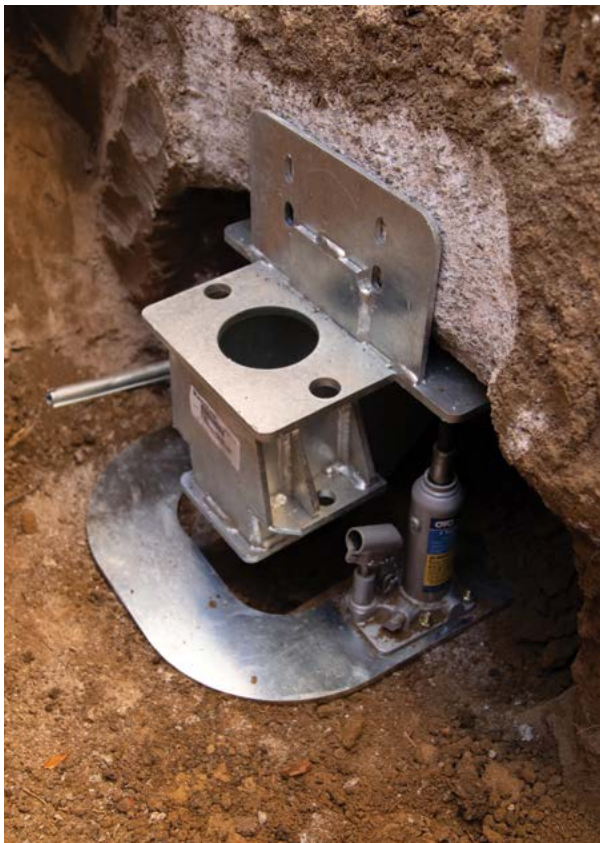
Figure 2.23 Bracket RAYser support system
