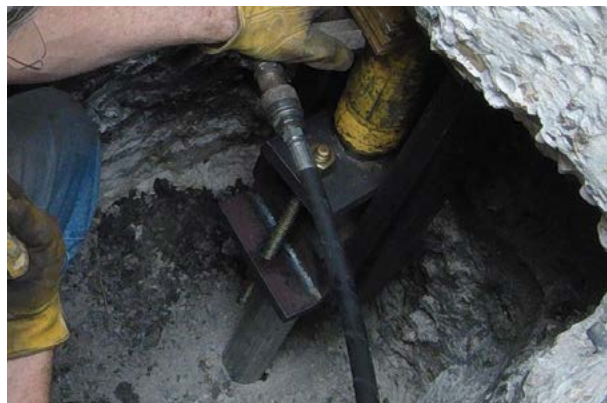
Figure 2.56 Place hydraulic cylinder and snug bracket against footing
