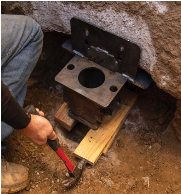
Figure 2.22 Temporary bracket support with wood cribbing
