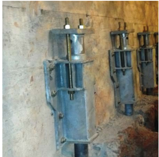
Figure 2.45 Flush-mount bracket installation
