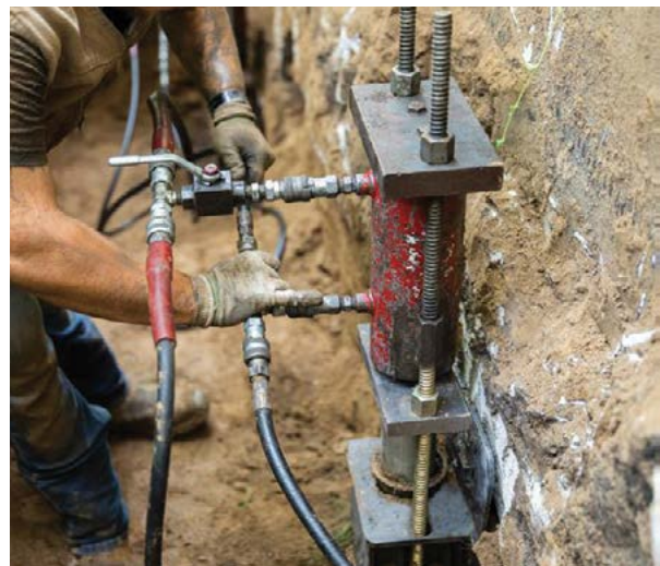
Figure 2.39 Connection of lift cylinder assembly
