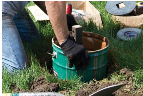
Figure 1.103 Setting the reservoir
