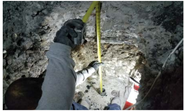
Figure 2.53 Measure from bottom of footing to top of installed pier section
