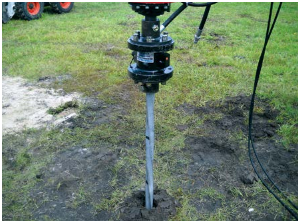
Figure 1.85 Shaft twist
