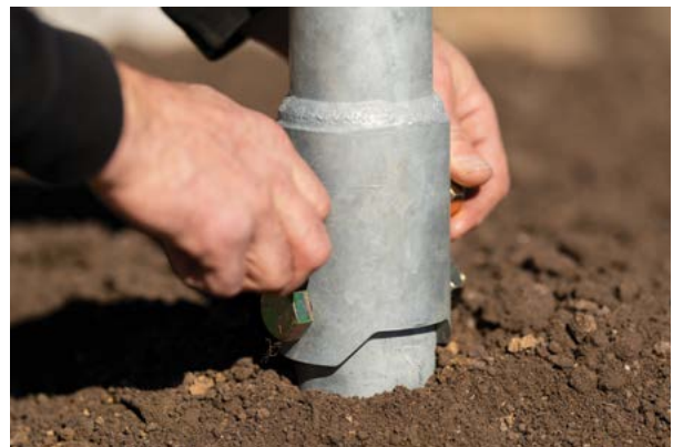
Figure 1.88 Install coupler bolts
