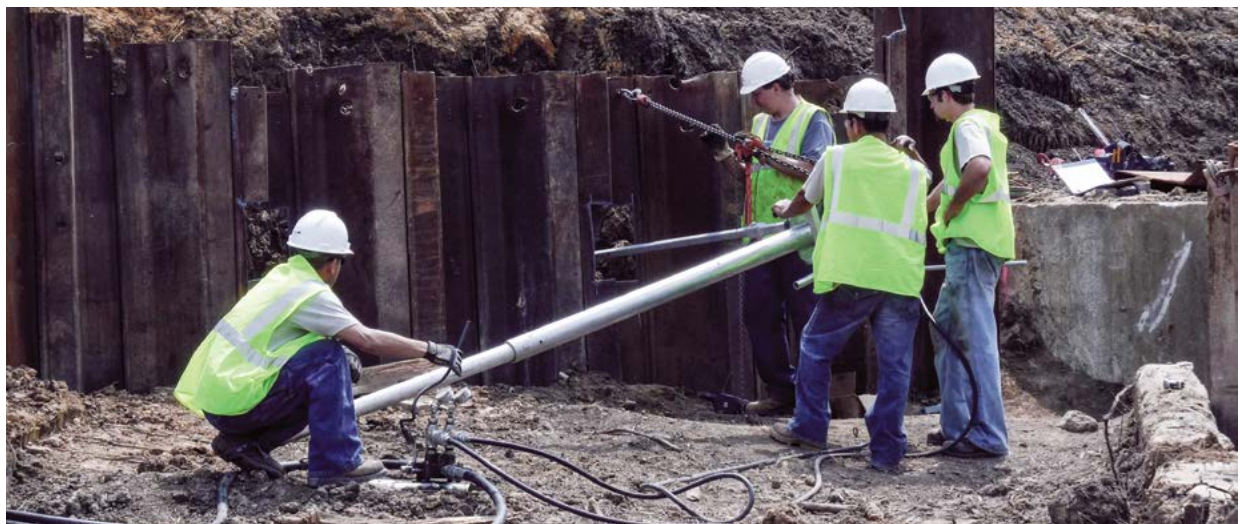
Figure 1.77 Torque arm
