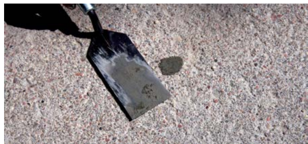
Figure 5.18 Patching the injection hole
