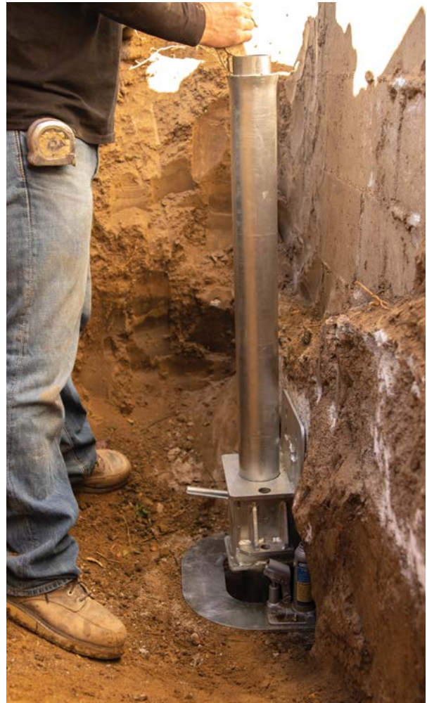
Figure 2.25 Sleeve and starter inserted together through the bracket
