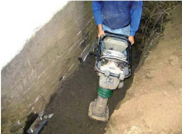
Figure 2.43 Backfill excavations and compact soil
