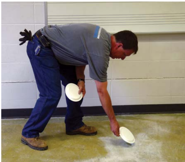
Figure 2.63 Marking slab pier locations
