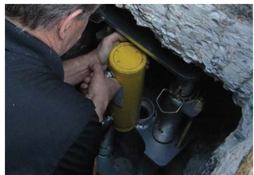
Figure 2.50 Placement of hydraulic drive cylinder
