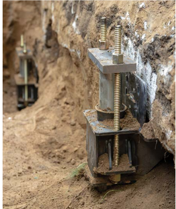
Figure 2.41 System locked off; pier installation complete
