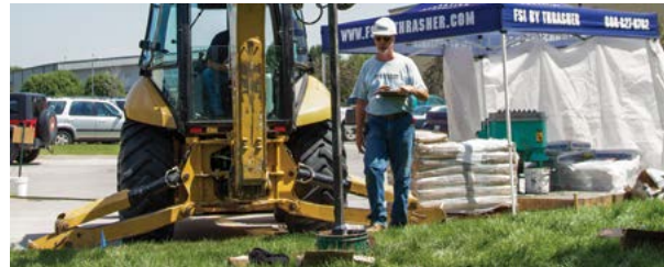
Figure 1.98 Grout mixing station near work area
