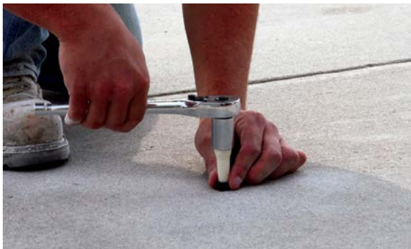
Figure 5.16 Injection port tightened with a socket wrench
