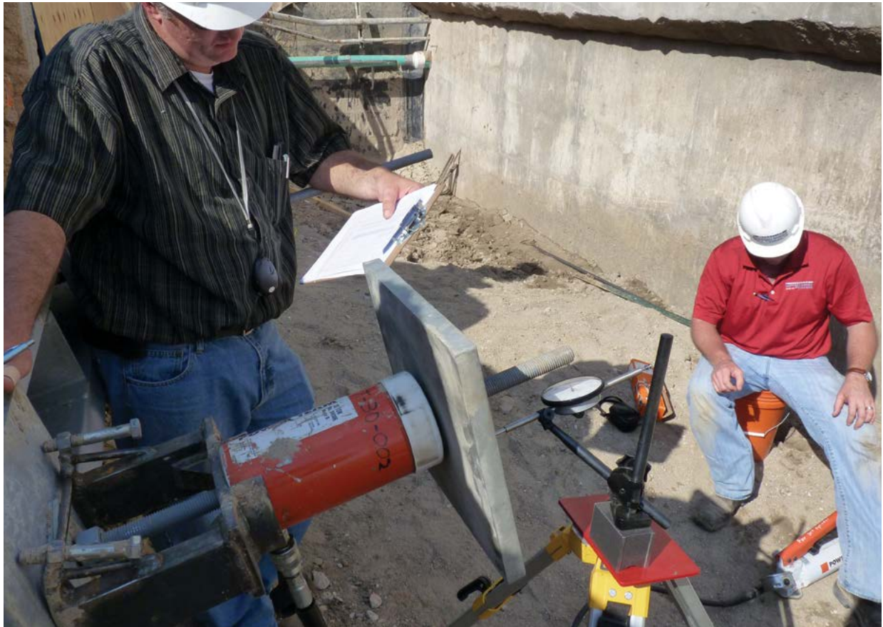
Figure 1.49 Pretensioning helical tieback
