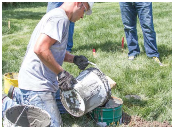
Figure 1.104 Pouring grout into the reservoir
