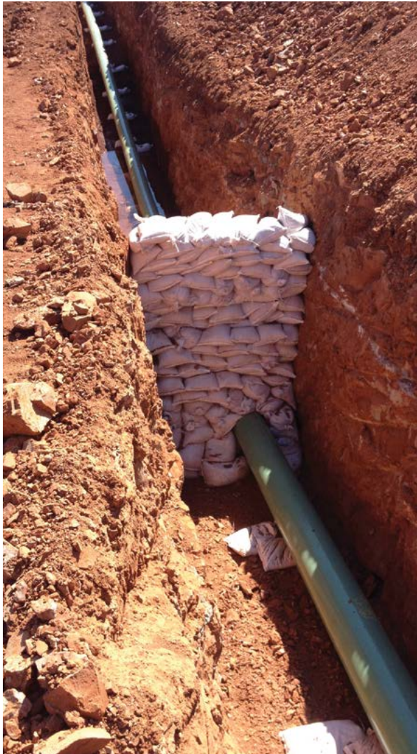
Figure 5.9 Sandbag trench breaker for pipeline
