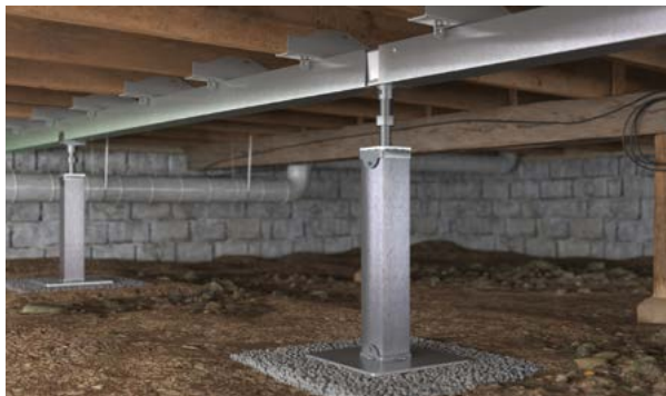
Figure 4.1 Rendering of Model 350 SmartJacks providing supplemental support for joists in a crawl space
