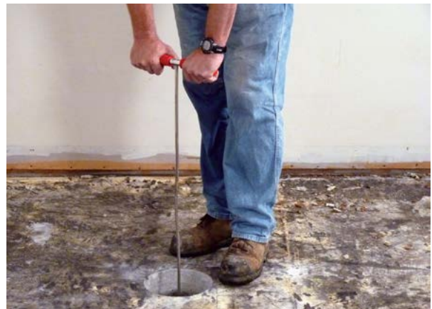
Figure 2.66 Probing for utilities or obstructions
