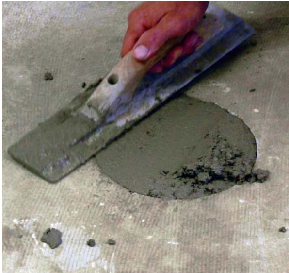
Figure 2.82 Patching holes at pier locations
