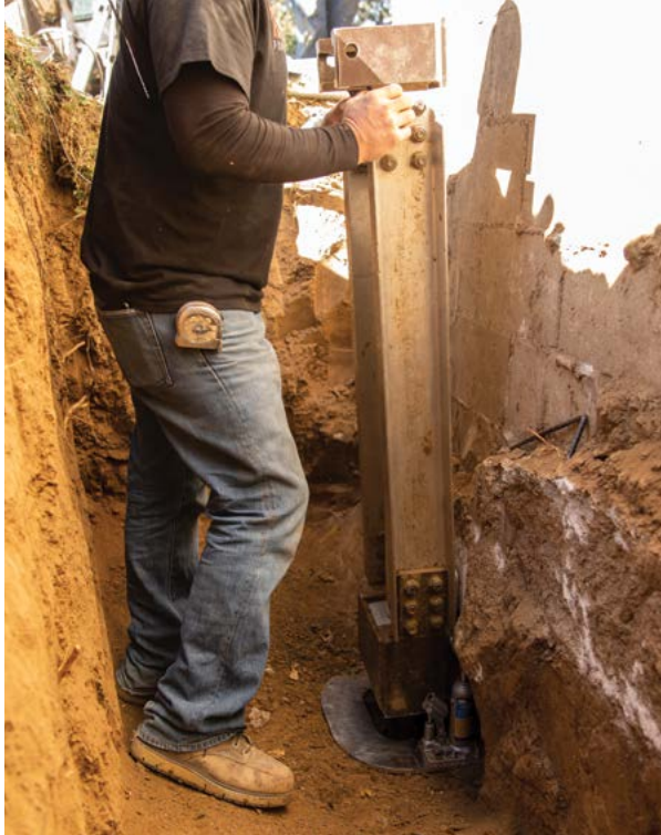
Figure 2.26 Drive stand for PP288 push pier system fitted to the bracket
