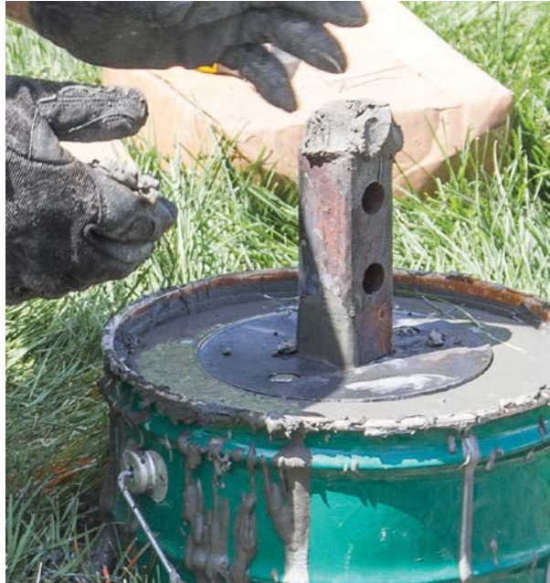
Figure 1.112 Buttering the top of the extension
