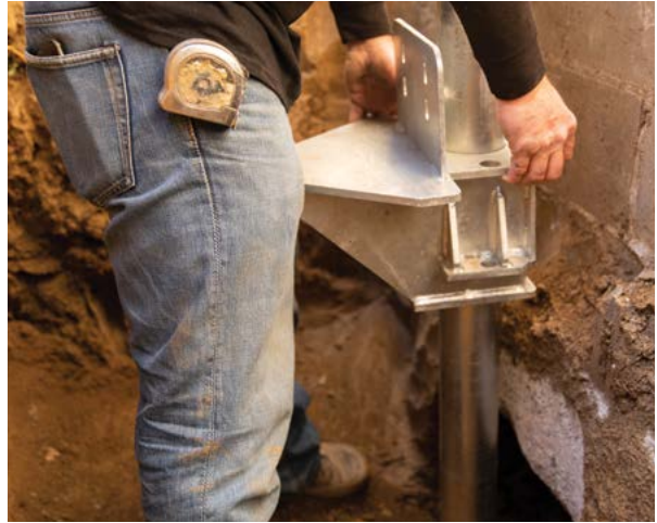
Figure 1.93 Lower assembly over pile shaft
