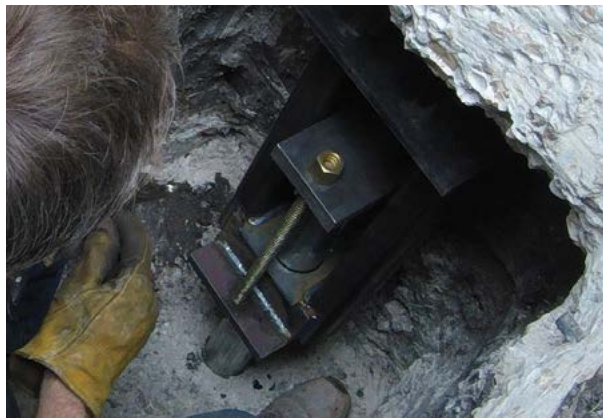
Figure 2.55 Place bracket assembly onto last driven pier tube
