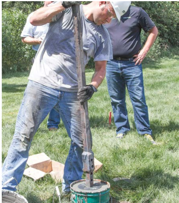
Figure 1.113 Placing an additional extension
