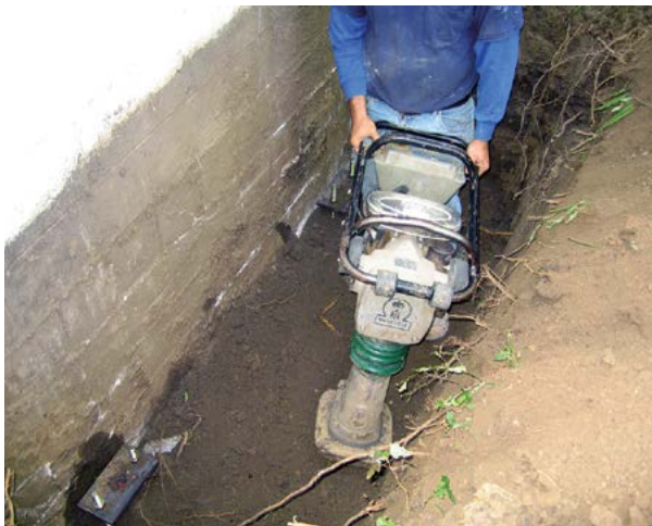
Figure 1.97 Backfill and compact soil
