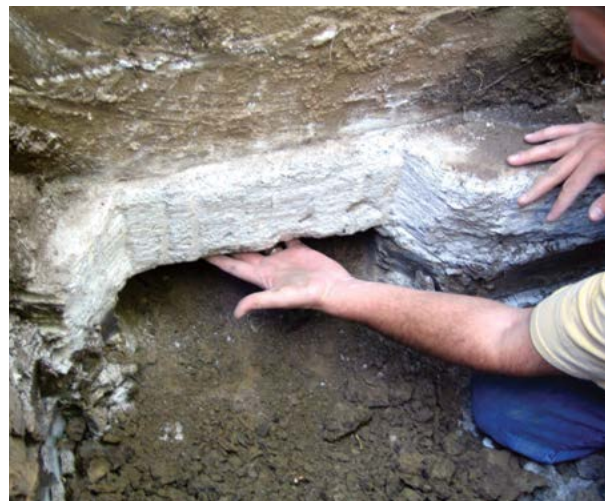
Figure 2.20 Checking underside of footing for proper preparation
