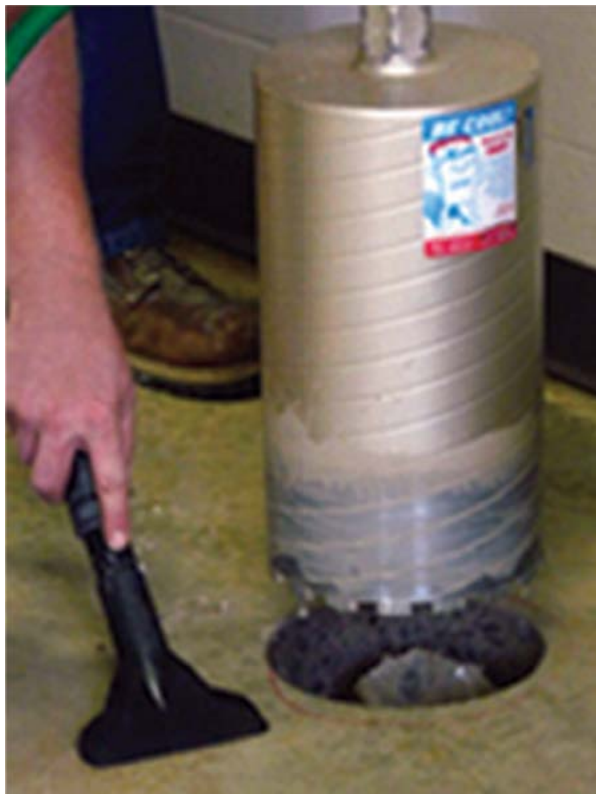
Figure 2.65 Concrete coring
