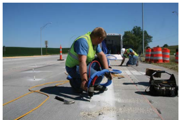
Figure 5.12 Monitoring pavement lift with string lines
