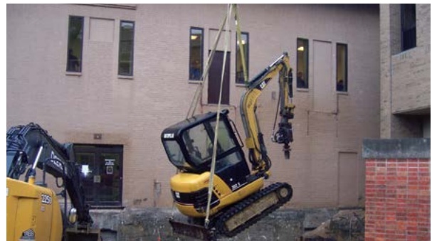
Figure 1.33 Mini-excavator lowered by crane into excavation to install helical tiebacks
