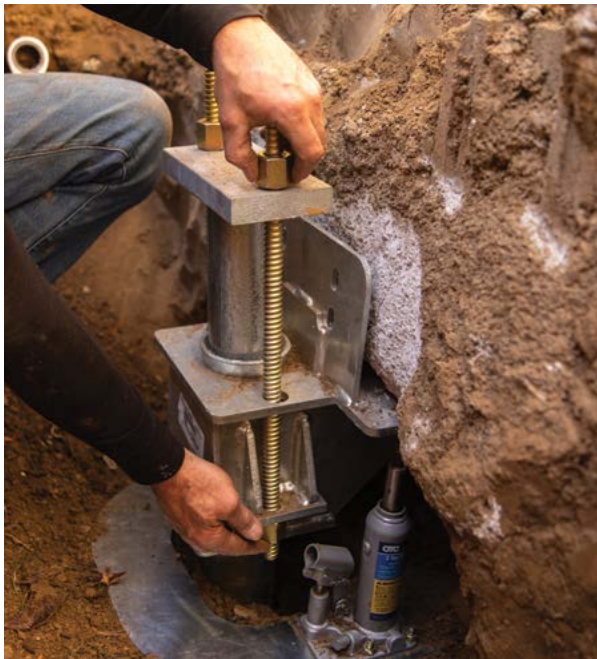
Figure 2.37 Installation of pier cap plate with coil rods and nuts
