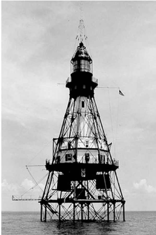
Figure 1.1 Lighthouse supported by screw (helical) pile foundations
