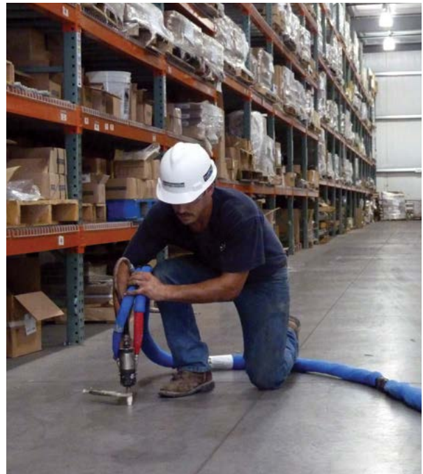
Figure 5.6 PolyLevel stabilizes warehouse floor slab
