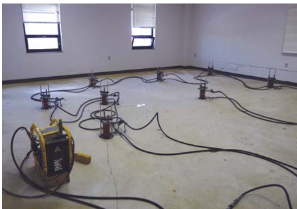
Figure 2.79 Lift cylinders connected for simultaneous loading
