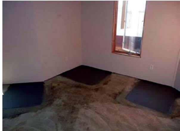
Figure 2.44 Concrete placement at interior pier locations
