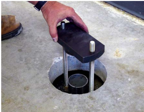
Figure 2.74 Pier tube cut to length; pier cap placed
