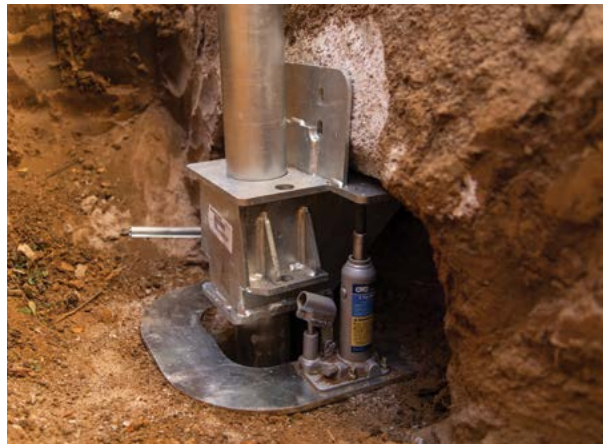
Figure 1.94 Bracket RAYser™
