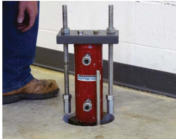
Figure 2.76 Lift cylinder assembly set on pier cap
