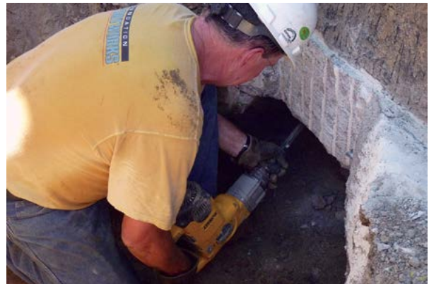
Figure 1.91 Footing preparation
