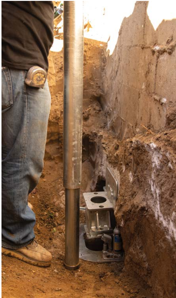
Figure 2.24 Exterior sleeve slid over the starter tube
