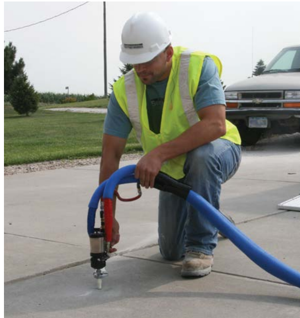
Figure 5.17 PolyLevel foam injected below the slab
