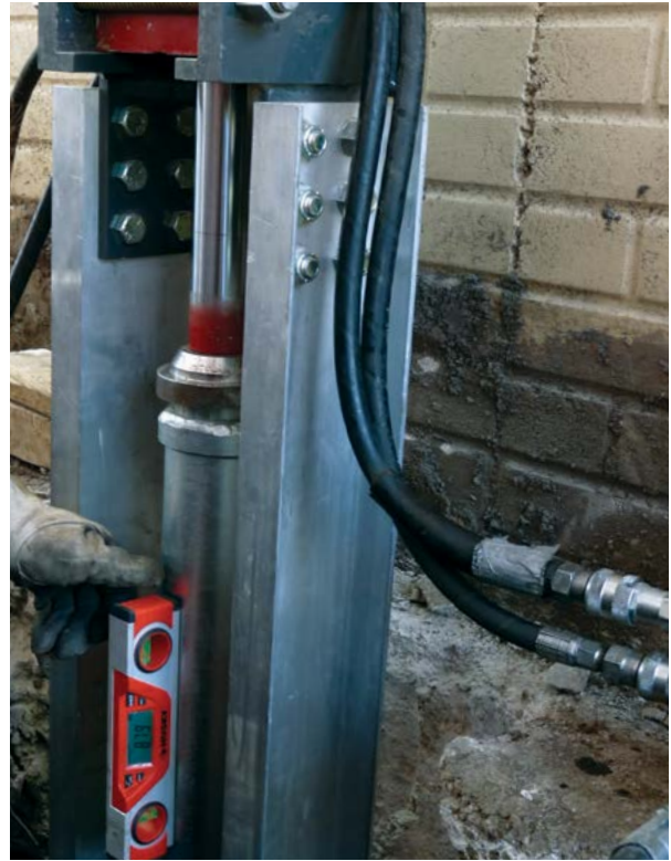
Figure 2.31 Checking drive stand alignment with digital level
