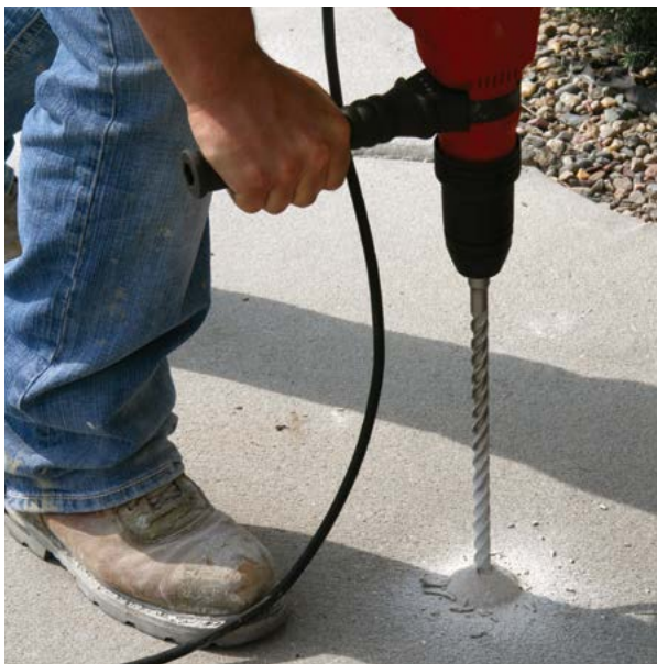
Figure 5.15 Concrete slab drilled to provide access holes
