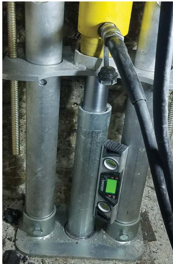
Figure 2.52 Check alignment of drive stand and starter section
