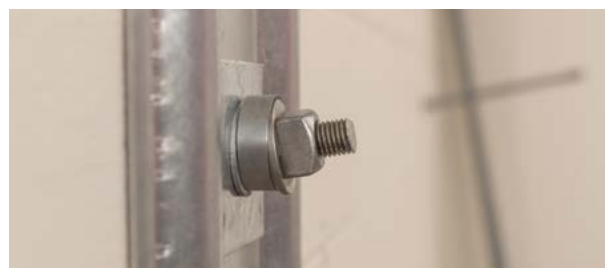
Figure 3.16 Hemispherical washer
