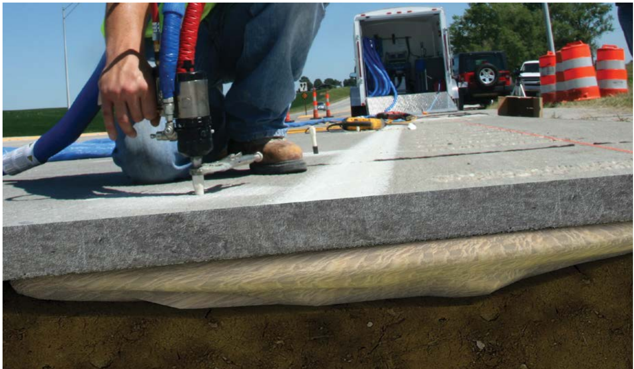
Figure 5.1 Rendering of PolyLevel foam injection beneath concrete pavement
