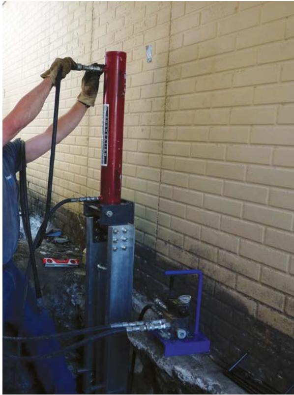
Figure 2.30 Connect hydraulic hoses
