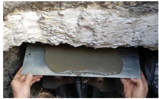
Figure 2.48 Grout plate used to create uniform bearing
