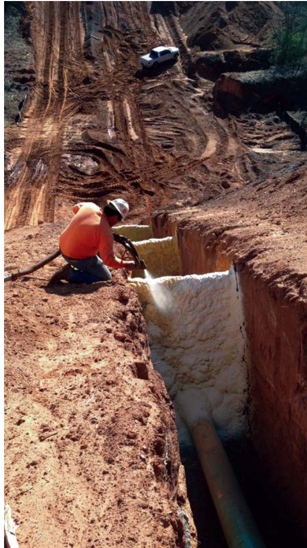
Figure 5.10 Placement of polyurethane foam trench breaks
