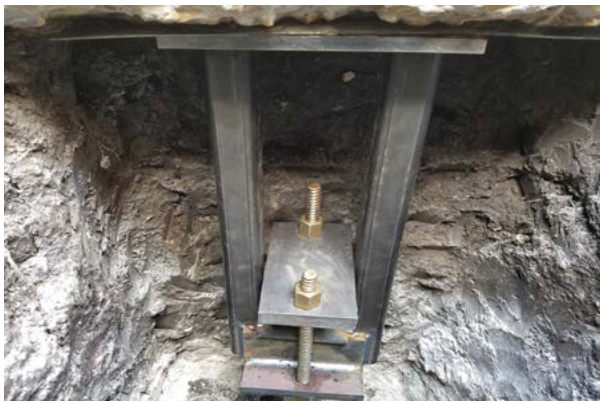
Figure 2.57 Completed concentric pier installation
