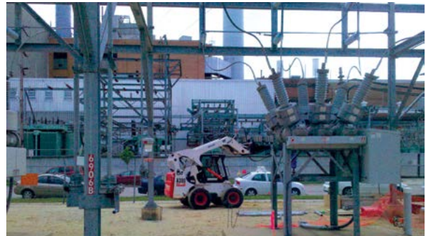
Figure 1.32 Skid steer installing helical piles within limited space at a substation
