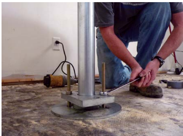
Figure 2.71 Slab pier drive adaptor installed
