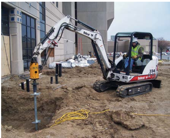
Figure 1.3 New construction helical pile installation
