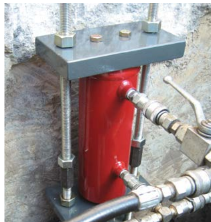
Figure 2.12 Foundation Supportworks FS35LCA lift cylinder assembly
