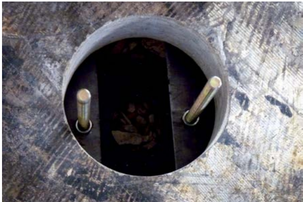
Figure 2.69 Threaded rods installed
