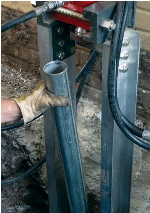
Figure 2.33 Installing PP288 push pier tube
