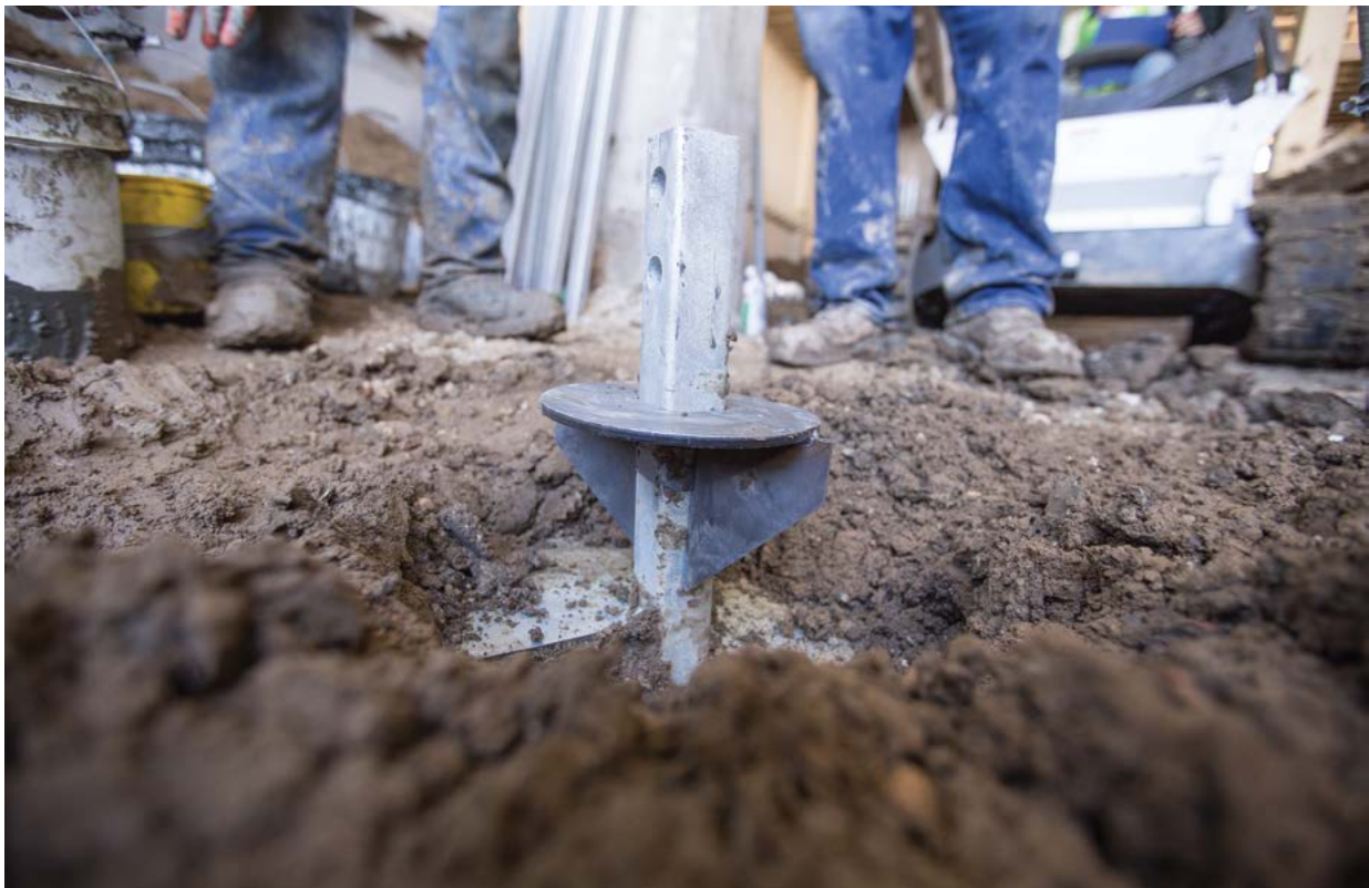
Figure 1.60 Spiked Lead Displacement Plate
