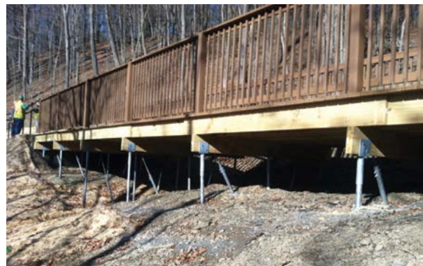
Figure 1.30 Boardwalk supported on 2.375" O.D. vertical and battered helical piles
