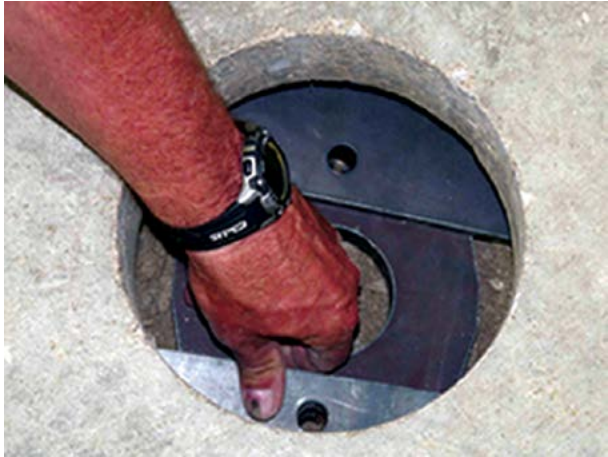
Figure 2.68 Main plate and wing plates positioned and aligned beneath the slab
