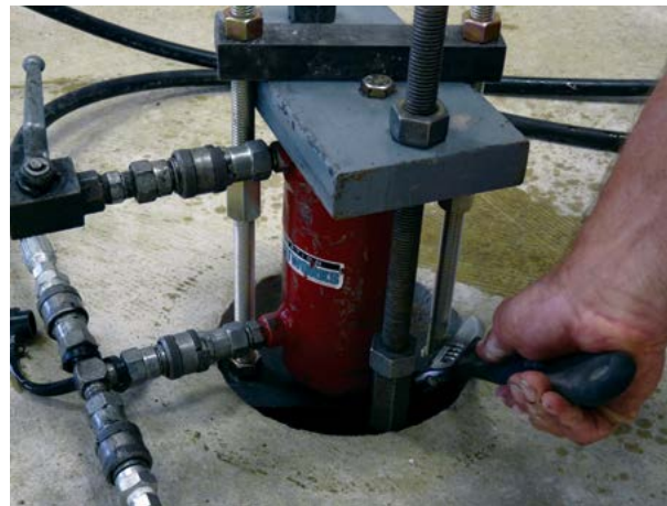
Figure 2.80 Pier load locked off by tightening nuts on top of pier cap
