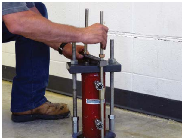
Figure 2.77 Lift plate assembly coupled to threaded rods of slab pier bracket
