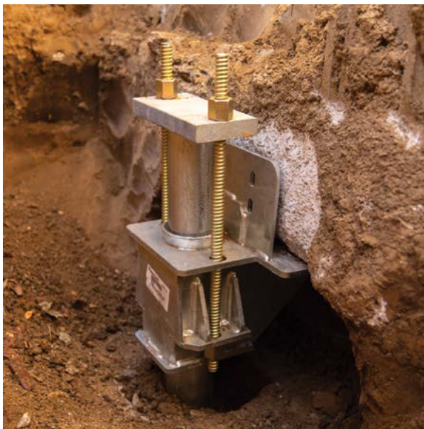
Figure 2.38 PP288 bracket ready for lift cylinder assembly
