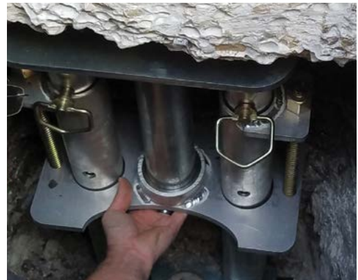
Figure 2.49 Drive stand setup within excavation
