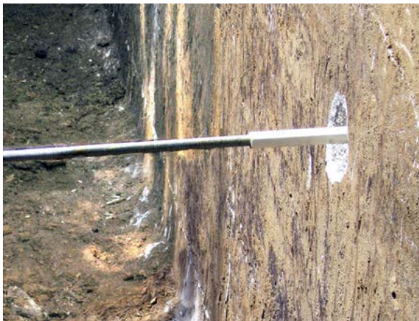
Figure 3.12 After: Shear movement recovered and wall stabilized with GeoLock anchors
