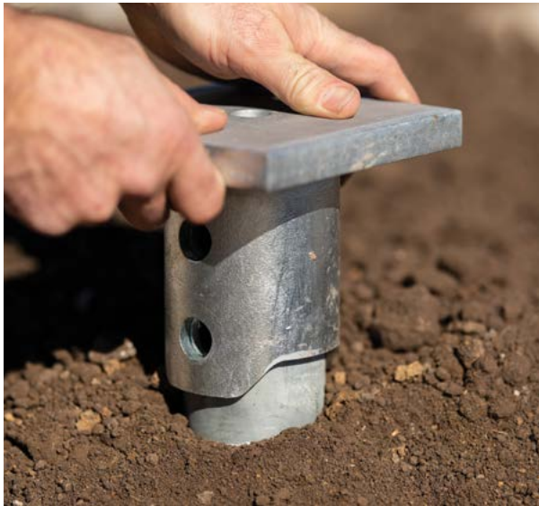
Figure 1.89 Install new construction bracket
