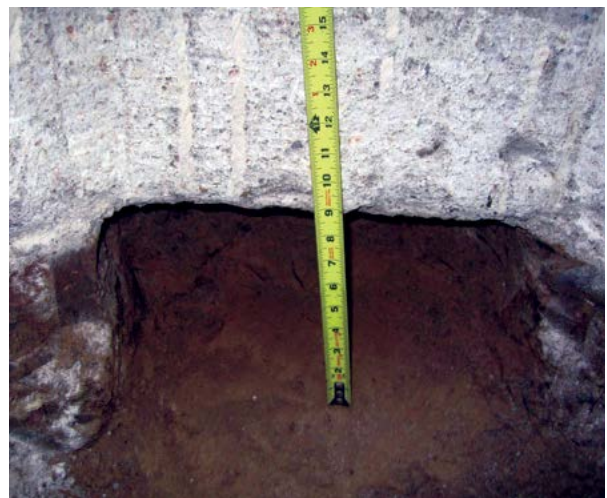
Figure 2.21 Completed footing excavation and preparation; ready to position bracket
