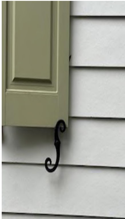
PAINTED WOOD BEVELED PANEL SHUTTER WITH OPERABLE HINGES, SHUTTER DOGS, AND BOLT
