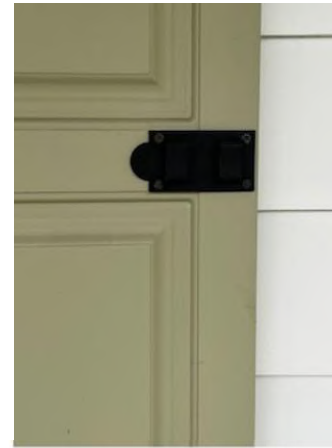
OPERABLE SHUTTER DOG AND BOLT
