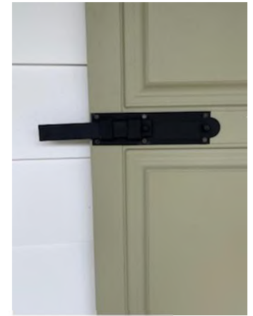
OPERABLE SHUTTER DOG AND BOLT
