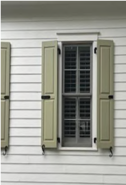
PAINTED WOOD BEVELED PANEL SHUTTER WITH OPERABLE HINGES, SHUTTER DOGS, AND BOLT
