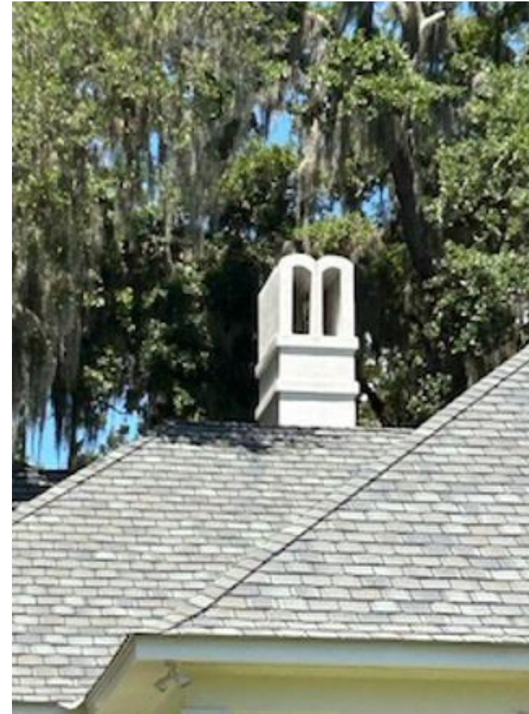
DOUBLE MASONRY CAP
