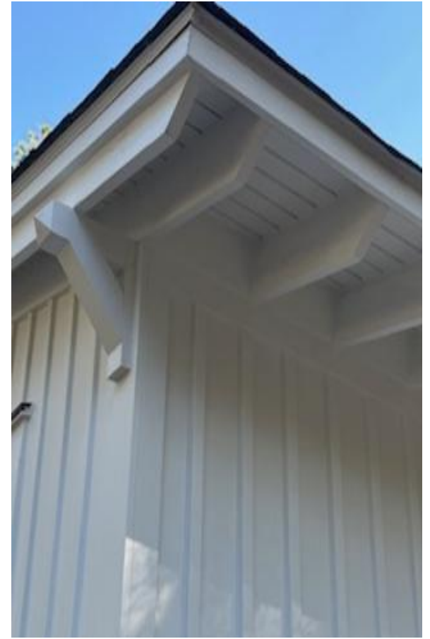
CORBEL AND OPEN RAFTER TAILS
