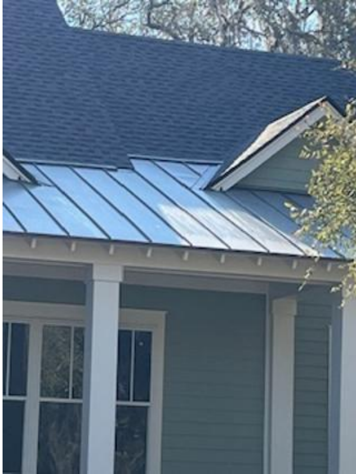
SHINGLE AND PAINTED METAL STANDING SEAM ROOF
